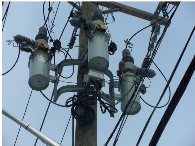
DTE is deploying triple single reclosers on the overhead circuits to isolate faults and remotely monitor current and voltage. The devices allow system supervisors increased ability to perform remote circuit switching to reduce outage time.
