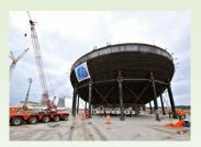
Vogtle Unit 3 Nuclear Island showing nuclear island basemat pour and Containment Vessel with exterior rebar installed (Courtesy of Southern Company)
