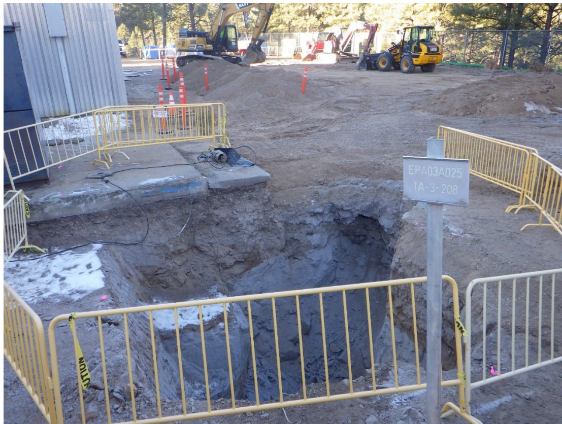
Deep excavation section (14.6 ft deep); excavation south of 14.6-ft section was backfilled prior to completing 14.6-ft section for safer access/operation - photo taken from above Outfall (EPA 03A025) looking southwest
