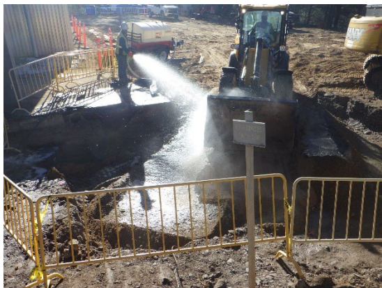
Backfilling the deep excavation section; dust suppression using water
