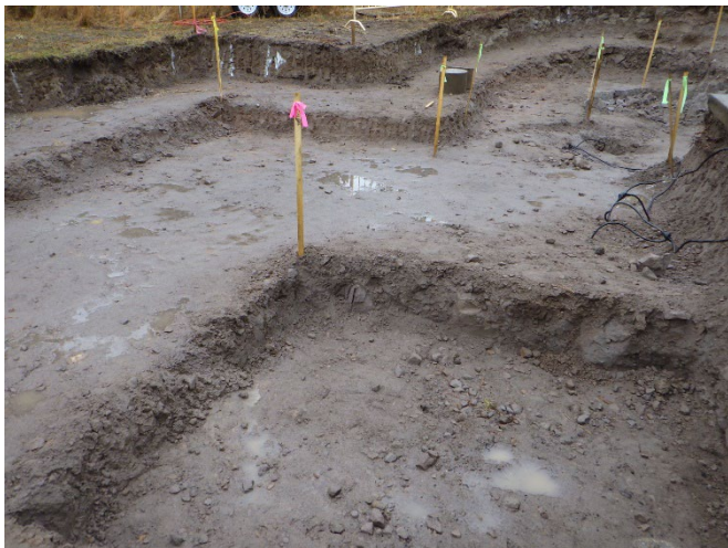
Excavation showing step down from 2-ft to 3-ft to 4-ft depth. Photo taken near SW corner of Transformer Pad (03-190) looking north
