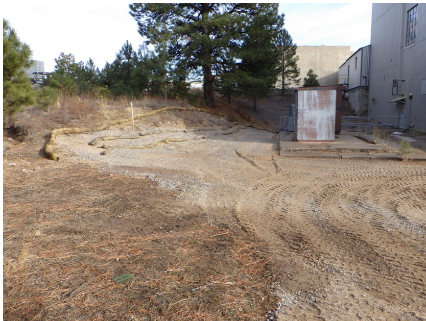
Photo taken from northwest side of excavation looking east
