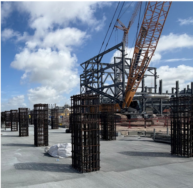
Photo 4: EFG Substation Foundation
