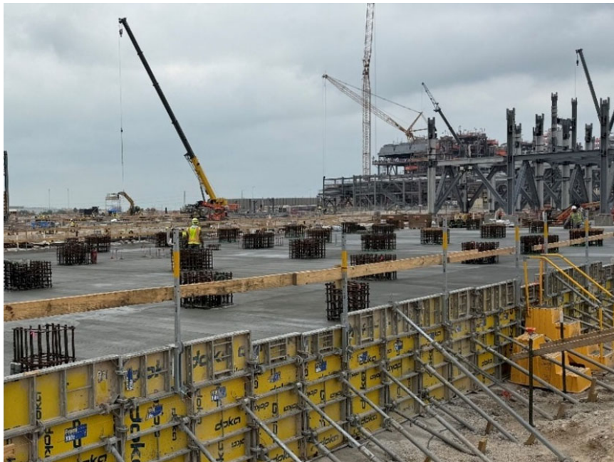
Photo 2: Train 8 Cryogenic Rack Foundation
