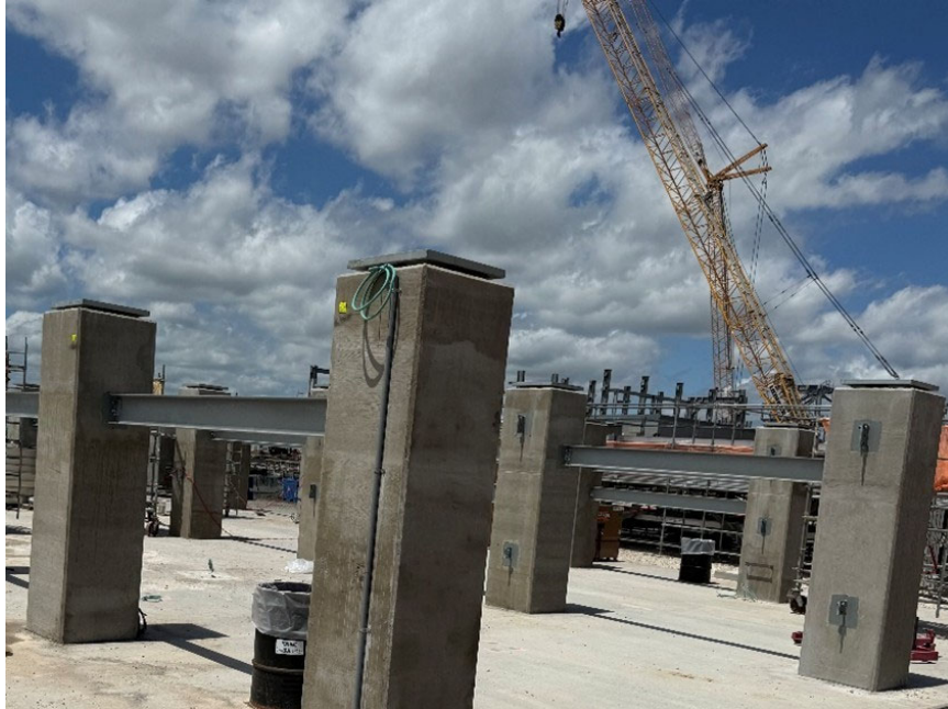
Photo 3: Train 8 Liquefaction Substation Pedestals
