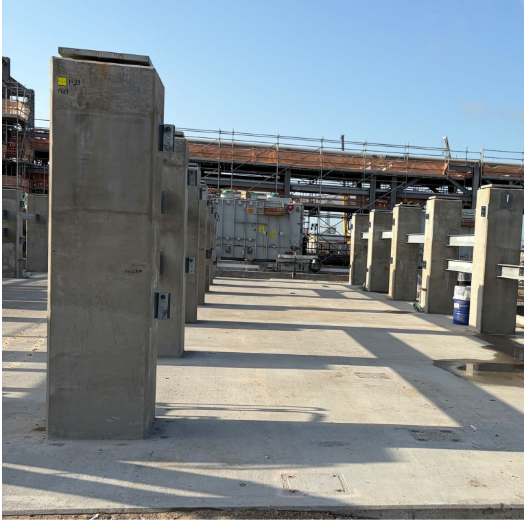
Photo 4: Train 8 Liquefaction Substation Pedestals
