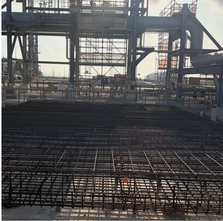
Photo 5: Refrigerant Storage Foundation
