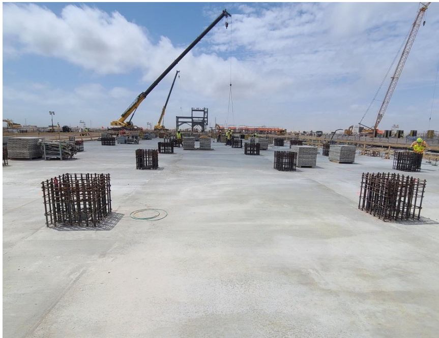
Photo 2: Train 8 Cryogenic Rack Foundation
