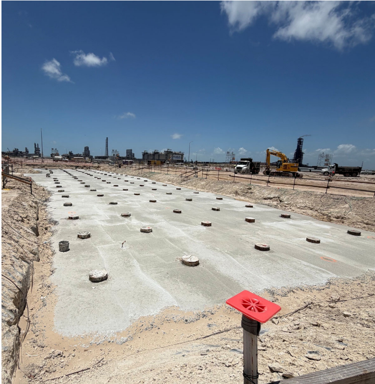
Photo 5: End Flash Gas Substation Foundation
