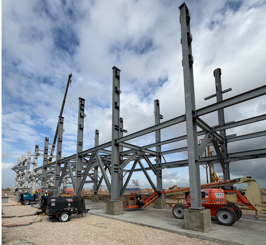
Photo 4: Train 8 Structural Steel
