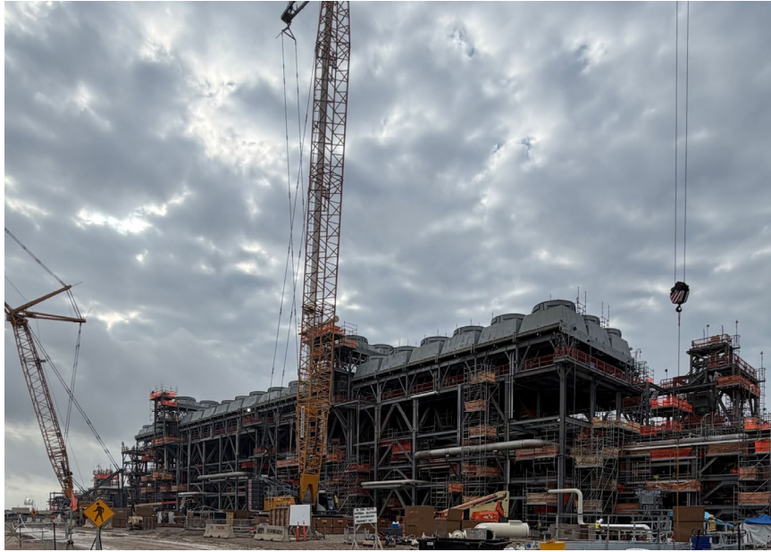
Photo 1: Train 7 Aboveground Piping Installation
