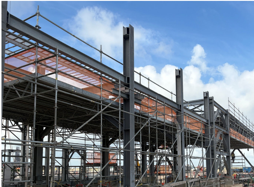
Photo 2: Train 8 Structural Steel
