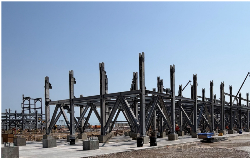
Photo 4: Train 8 Structural Steel
