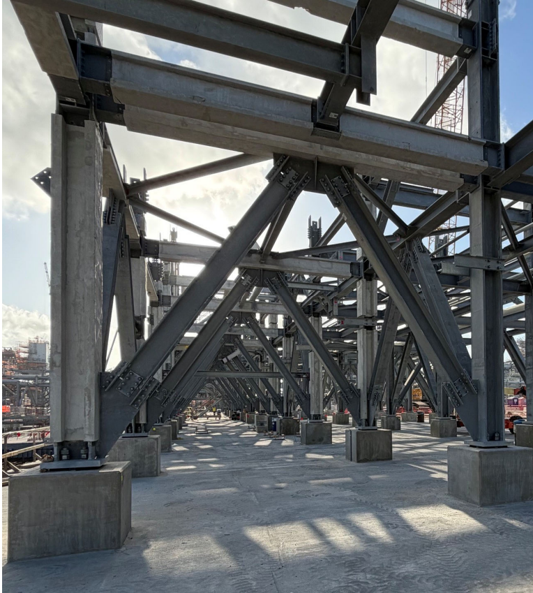
Photo 2: Train 8 Structural Steel
