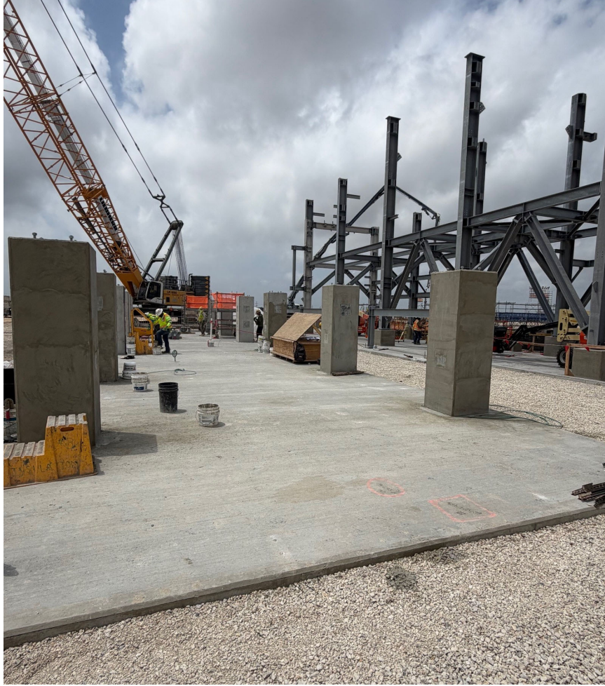
Photo 3: Train 8 Utility Substation Foundation
