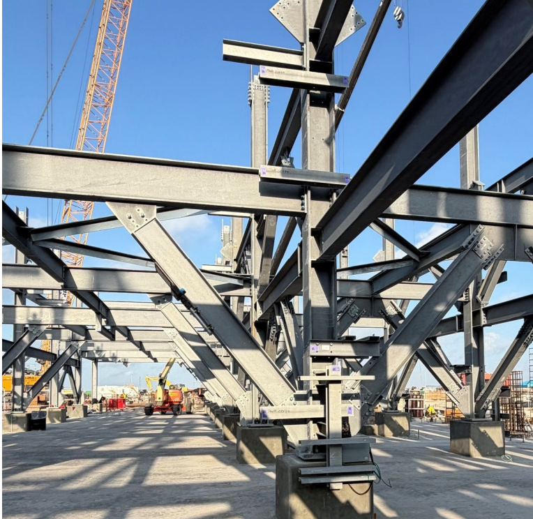
Photo 3: End Flash Gas Structural Steel
