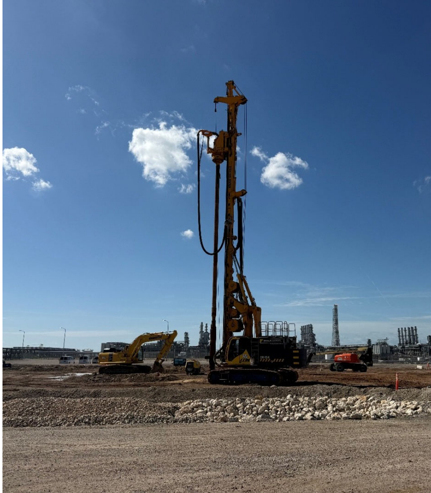
Photo 5: Refrigerant Storage Piling Installations
