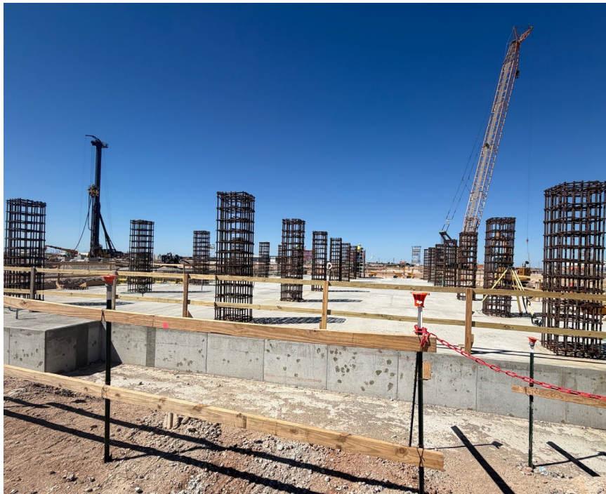
Photo 2: Train 8 Liquefaction Substation Foundation
