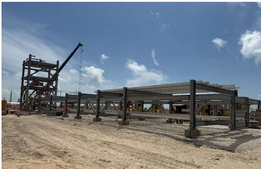
Photo 4: Train 8 Structural Steel
