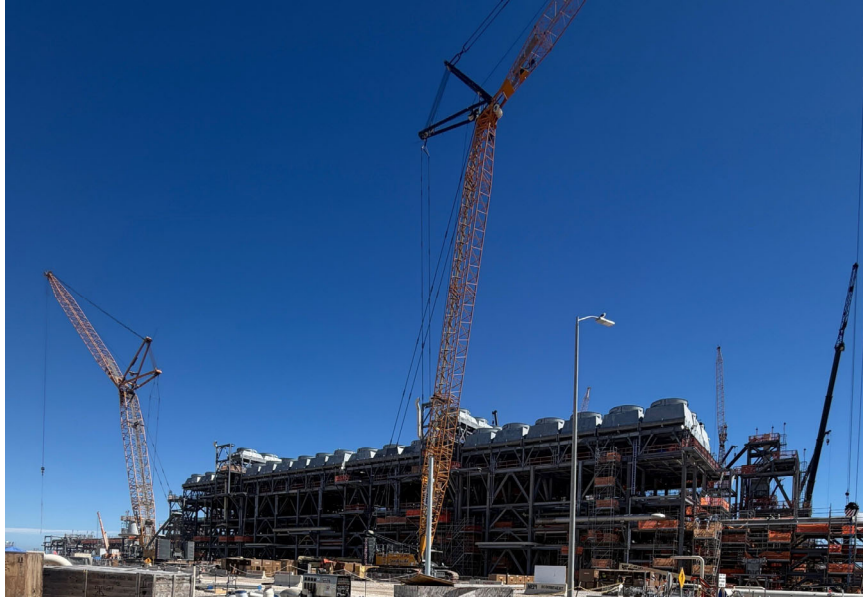
Photo 1: Train 7 Aboveground Piping Installation
