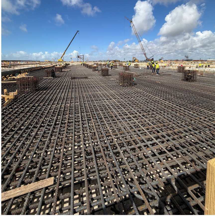
Photo 3: Train 8 Cryogenic Rack Foundation
