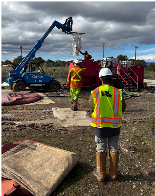
A DOE contractor prepares a batch of amendment for an injection as part of the pilot study at the Hazardous Materials Storage. Photo courtesy of CDM Smith.
