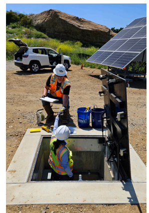
DOE contractors collect groundwater samples from a well connected to the solar-powered automated pump at the Former Sodium Disposal Facility. Photo courtesy of CDM Smith.
