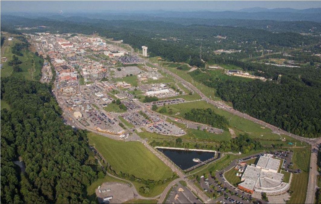
Y-12 National Security Complex
