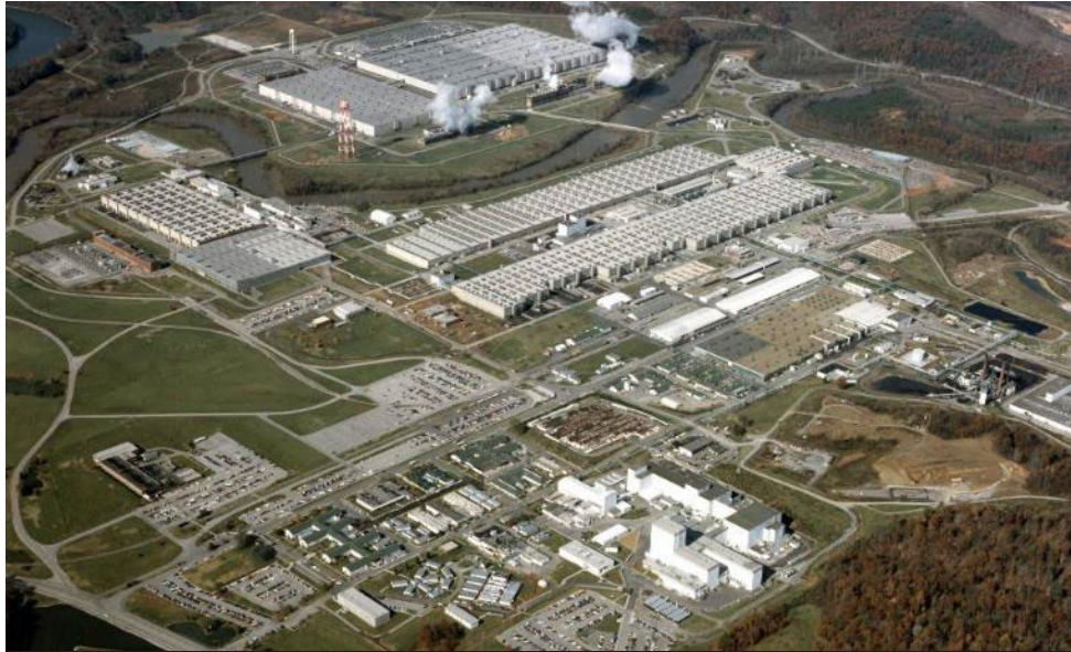
East Tennessee Technology Park before cleanup
