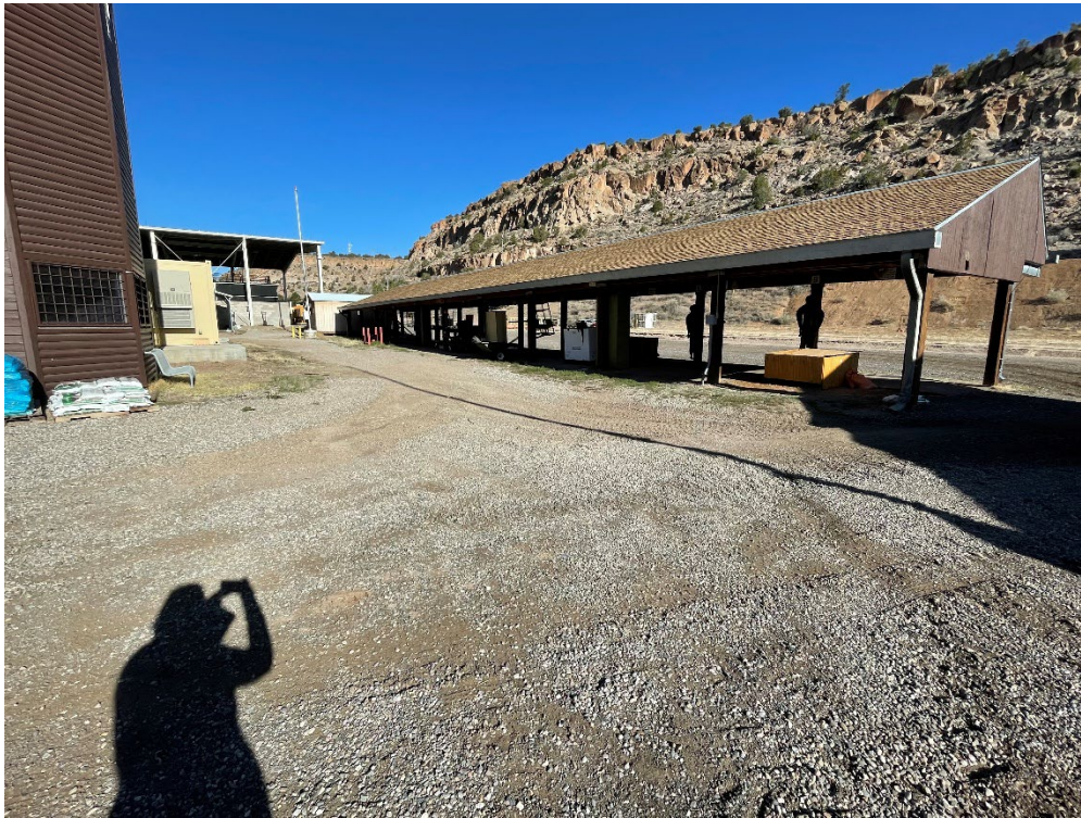
Figure 2. Proposed storage magazines location on the north side of Building 72-0091 looking northwest.
