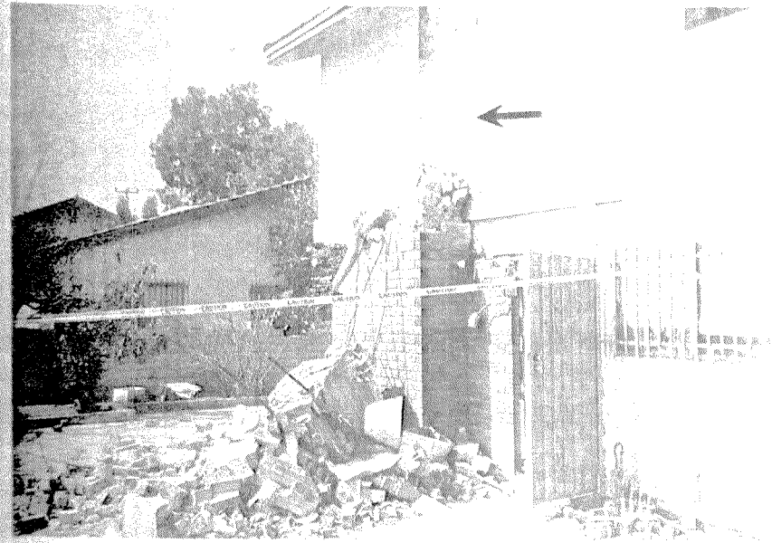
FIGURE 11.3 Collapse of brick chimney, 1994 Northridge, California, earthquake.
