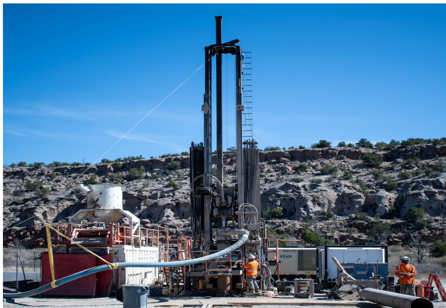
Drilling the R-80 groundwater monitoring well
