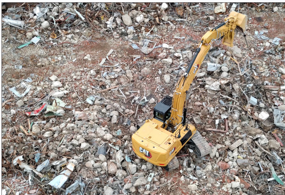
The Alpha-2 demolition project yielded 81 million pounds of debris and rubble.
