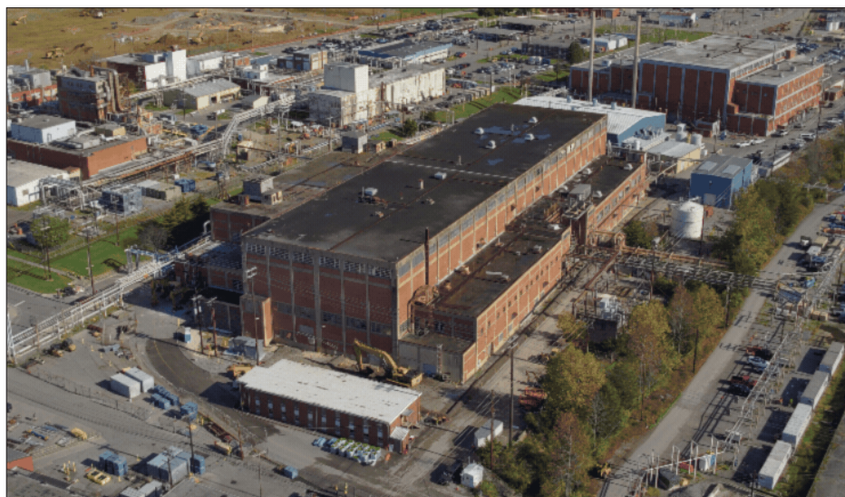
Teardown for Alpha-2 began in 2024 and was completed earlier this year, clearing 2.5 acres of land for reuse.
