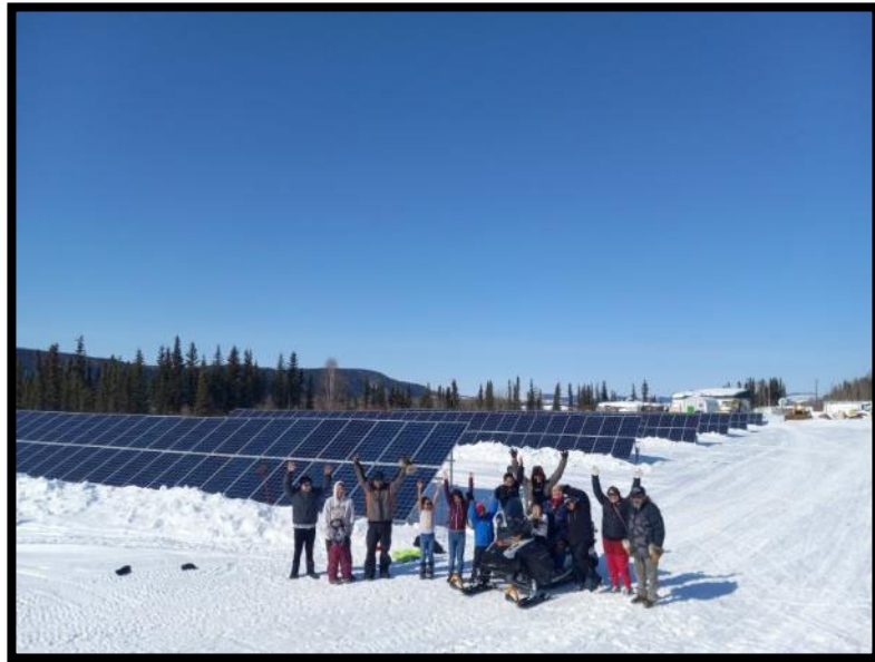
Hughes, Alaska Community Members in front of their solar array (source: https://www.energy.gov/oecd/energy-improvements-rural-or-remote-areas-selected-and-awarded-projects )
