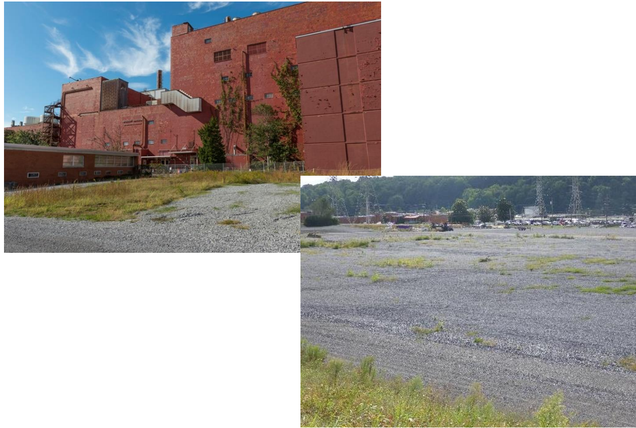
Biology Complex: Demolished February 2022
