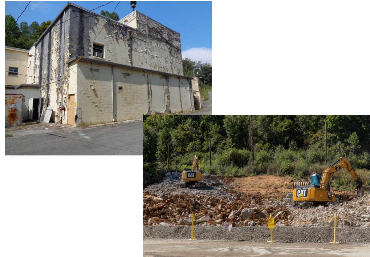
Building 9213 – Criticality Experimental Laboratory: Demolished December 2022
