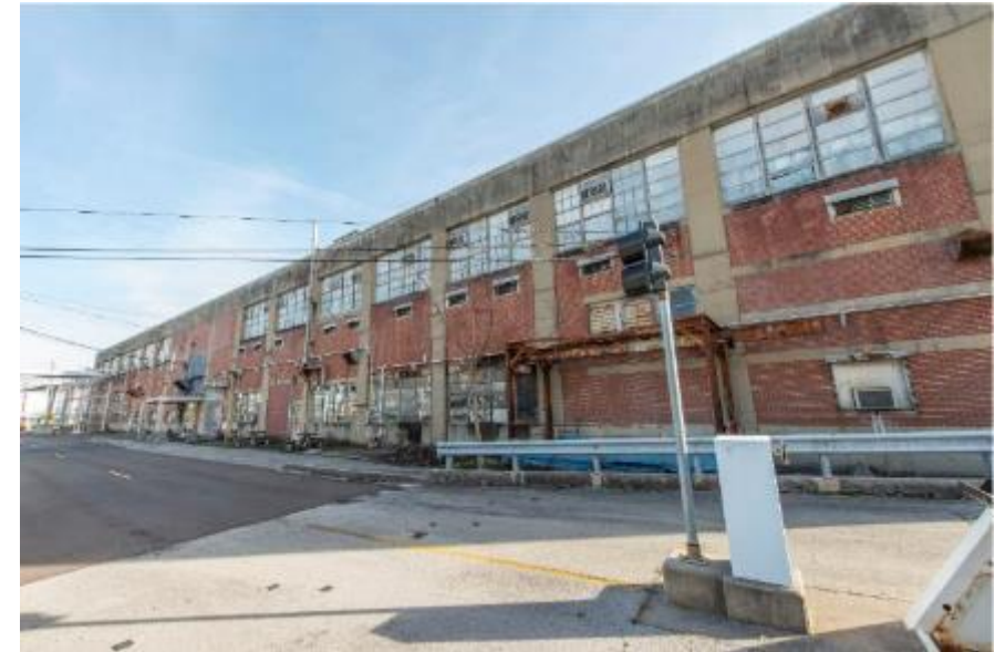
North Side of Beta-1 Facility
