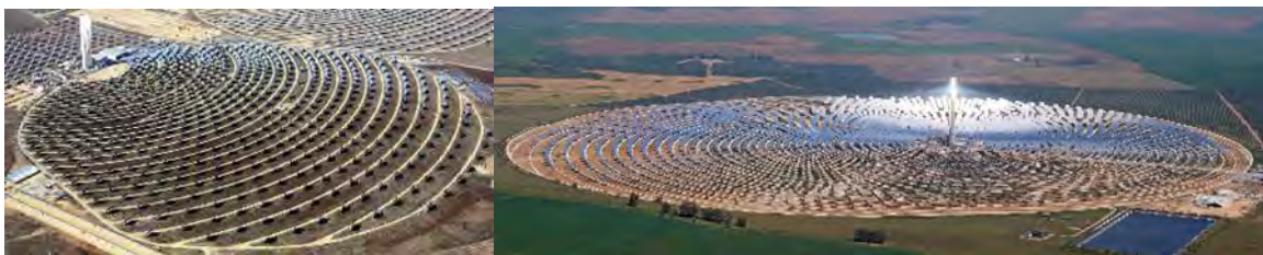
Figure A-43. Directional CSP System (PS-10) and Surround-Field CSP system (Gemasolar)
