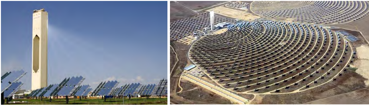
Figure A-42. Two Views of a Representative PV + CSP Solar Tower near Seville, Spain (PS-10), Which Has a Directional South-Facing (vs. Surround) Heliostat Field
