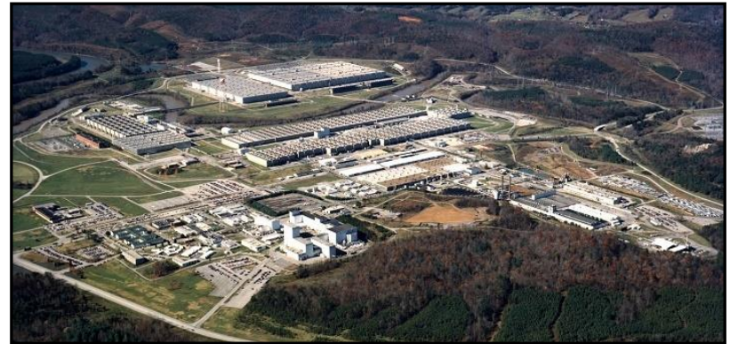
View in 1989 prior to cleanup
