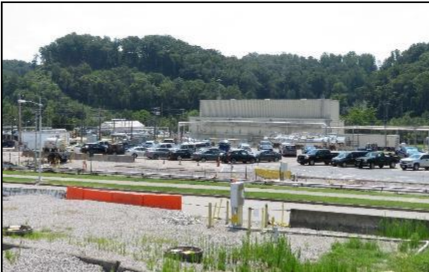
Parking area at former GAAT site
