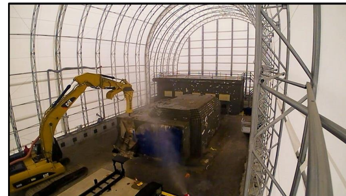
Demolition on the West Cell Bank
