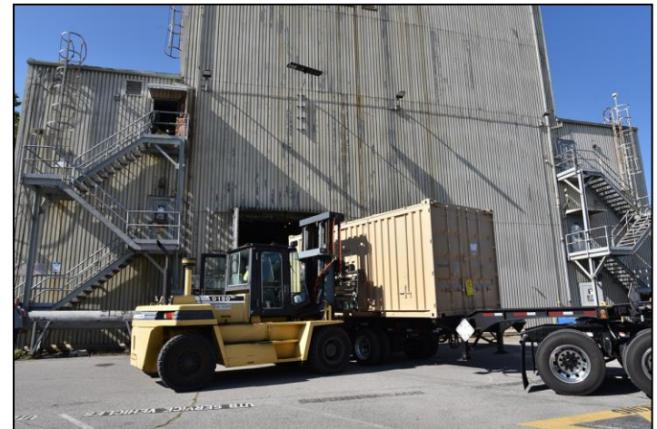
Teams remove waste from deactivation activities inside Building 3042
