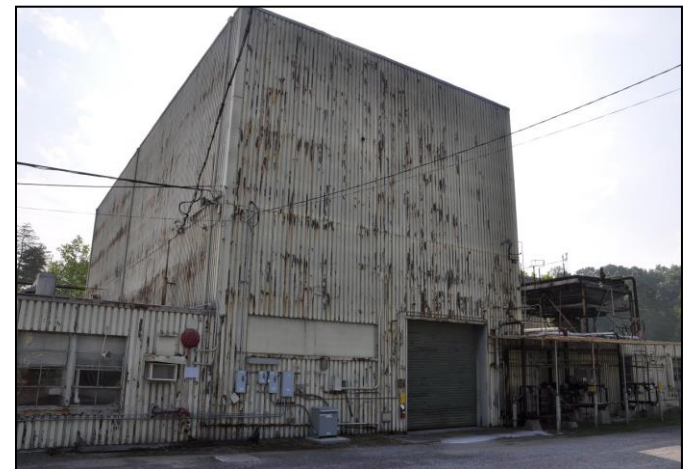
Building 7500 at ORNL
