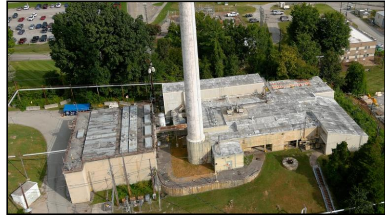
Aerial view of the Graphite Reactor support facilities
