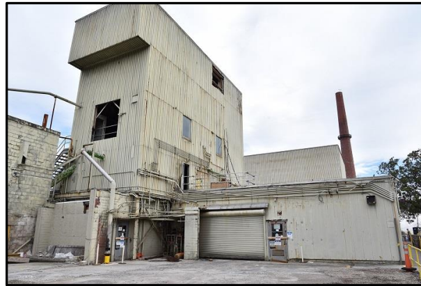
Building 3005 before major demolition
