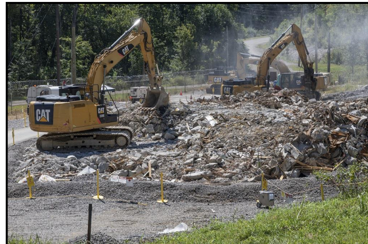
Crews finished demolition in 2022
