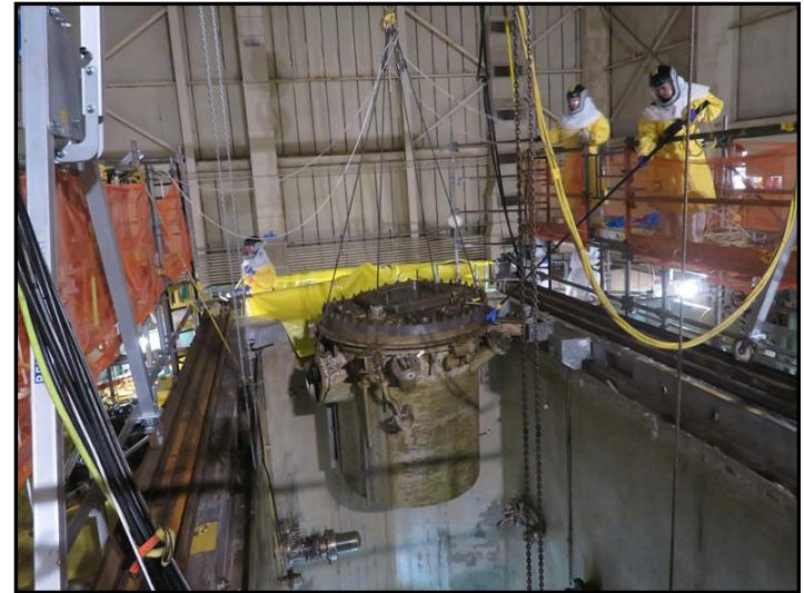
Crews lift and remove a portion of the reactor vessel
