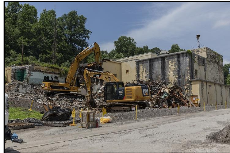
Demo underway on Building 9213
