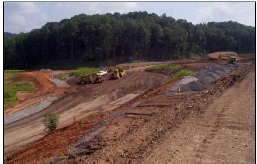
Remediation activities in 2005
