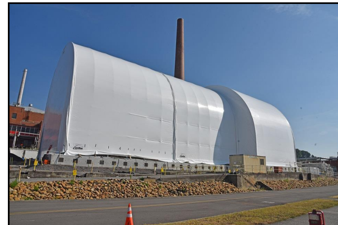
Building 3026 hot cells demolition enclosure
