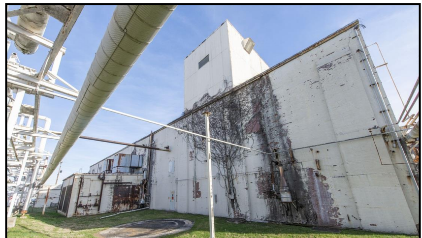
Building 9401-1 at Y-12
