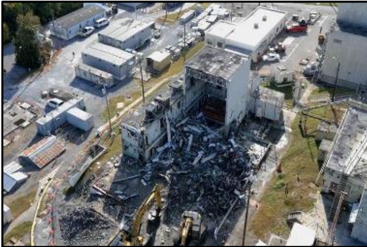
Bulk Shielding Reactor demolition
