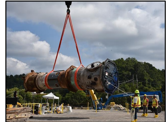
Removing the reactor vessel
