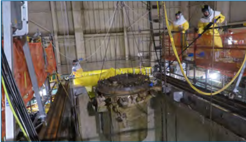
Removing the reactor vessel from the Oak Ridge Research Reactor
