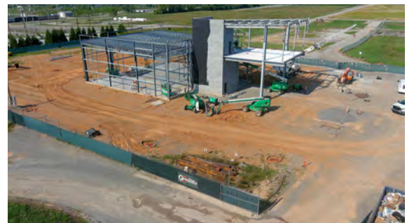
Construction progress on the K-25 Viewing Platform
