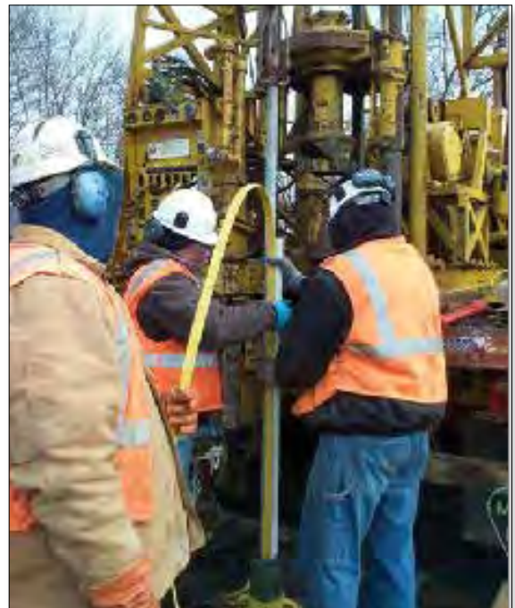
Monitoring wells were drilled on the west side of the Clinch River to determine if any contamination was migrating from DOE property into groundwater on private property
