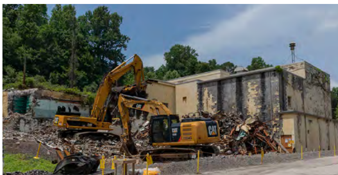
Crews demolish Building 9213
