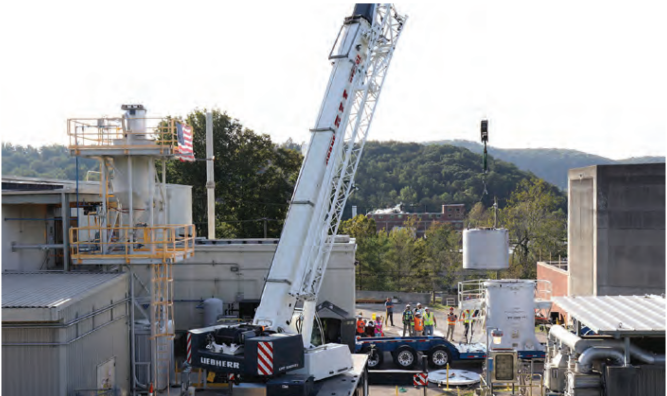
Workers load processed and downblended U-233 into a shipping cask for shipping and disposal.
