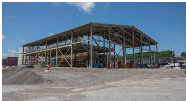
Construction progress on the treatment facility
