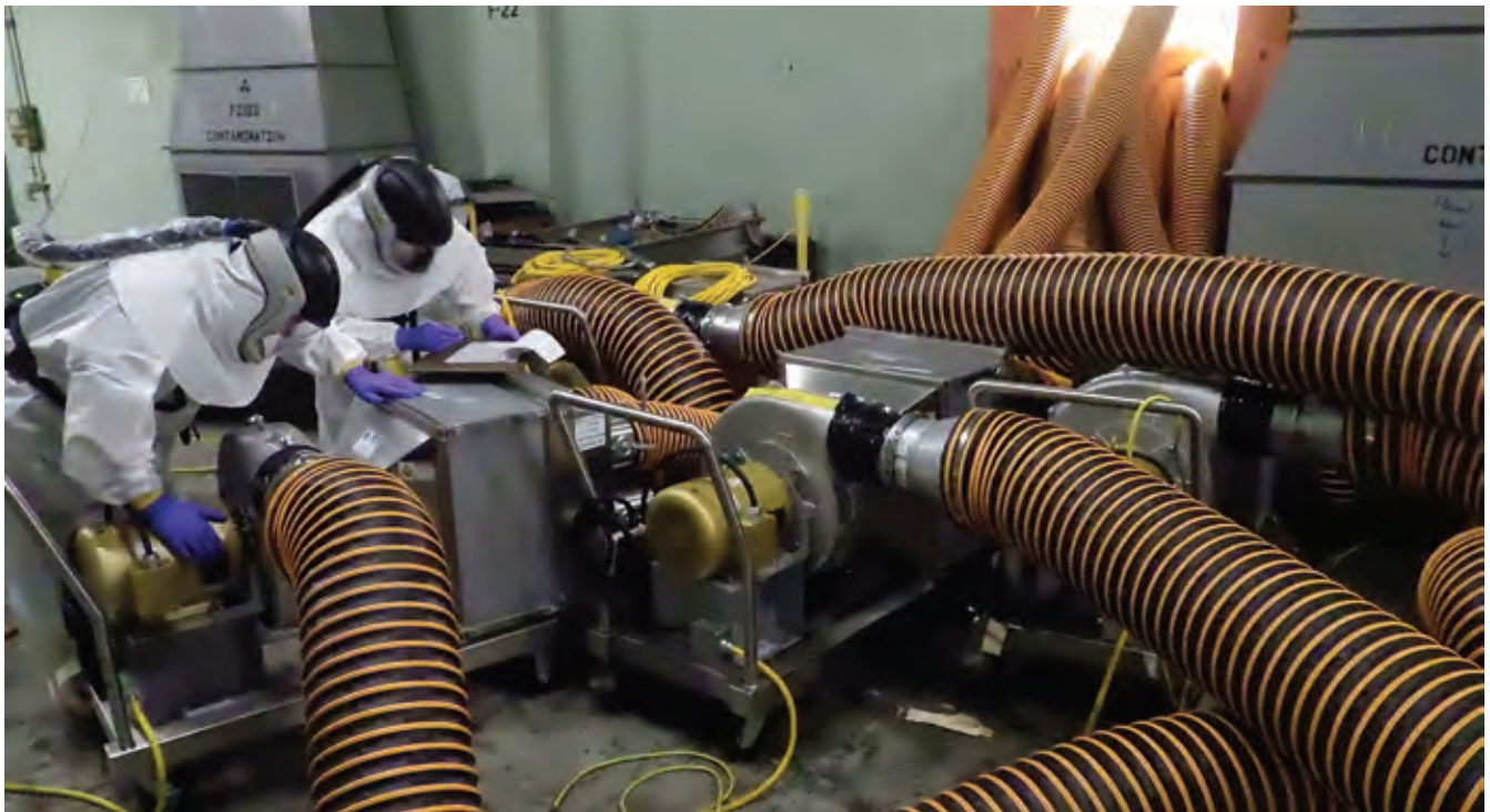
Air flow testing being conducted in Alpha-4
