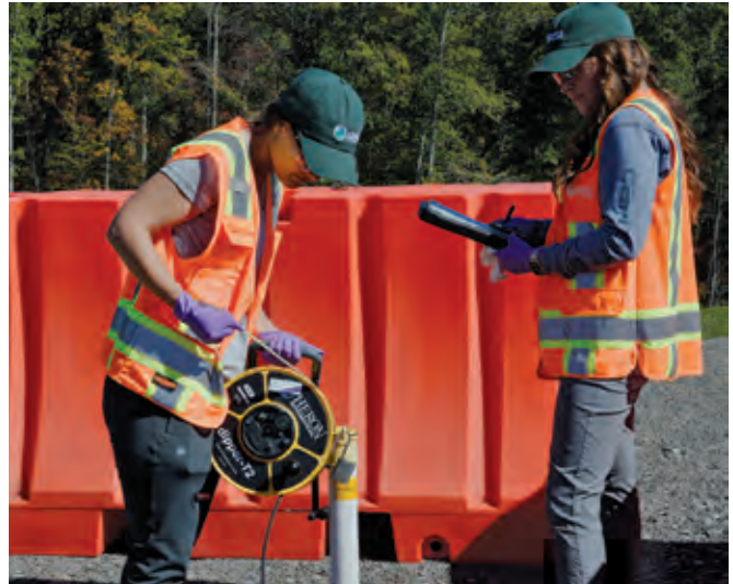
Workers perform groundwater monitoring at EMDF
