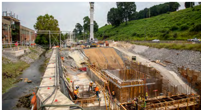
Construction progress on the headworks facility
