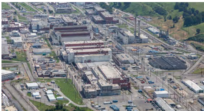
EM is tasked with demolishing numerous excess contaminated facilities, like these, at Y-12
