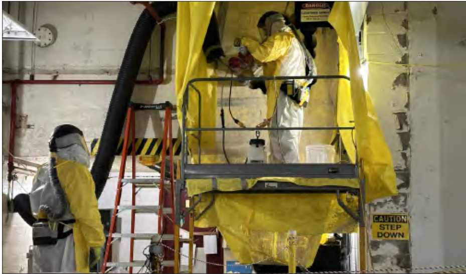
Workers perform deactivation activities inside Building 3003 at ORNL before demolition begins.
