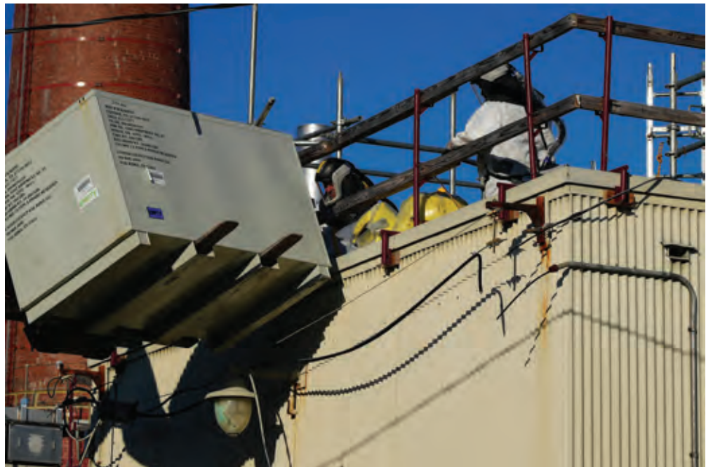
Waste being removed from an Isotope Row building
