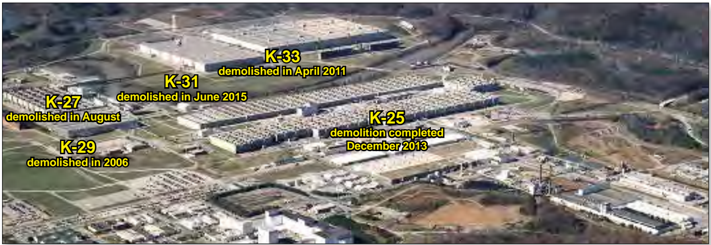
The K-25 Gaseous Diffusion Plant was renamed East Tennessee Technology Park in 1997. In 2020, OREM achieved its Vision 2020 goal of completing core cleanup at the site, which included demolishing more than 500 structures and addressing major areas of soil contamination. This is how the site looked before major demolition work began.
