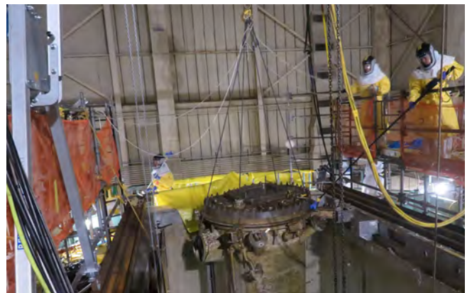
Teams remove the reactor vessel from the Oak Ridge Research Reactor
