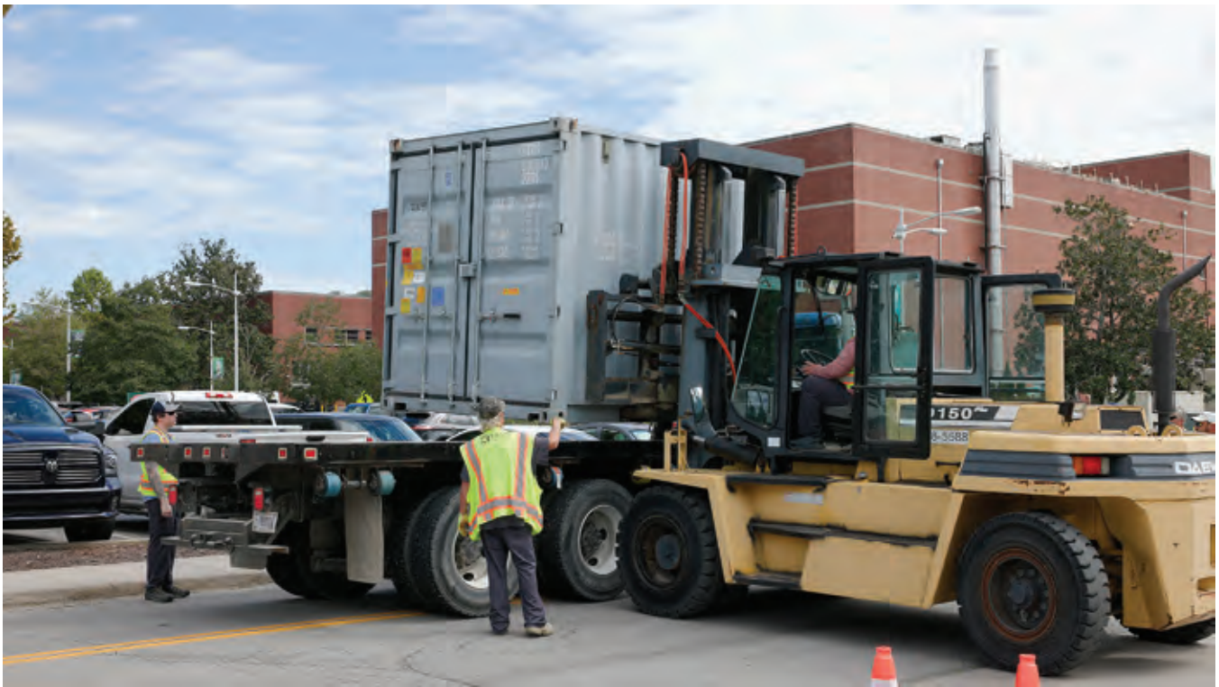
Workers remove a hot cell from Building 3038
