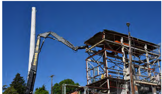
Workers take down the Low Intensity Test Reactor
