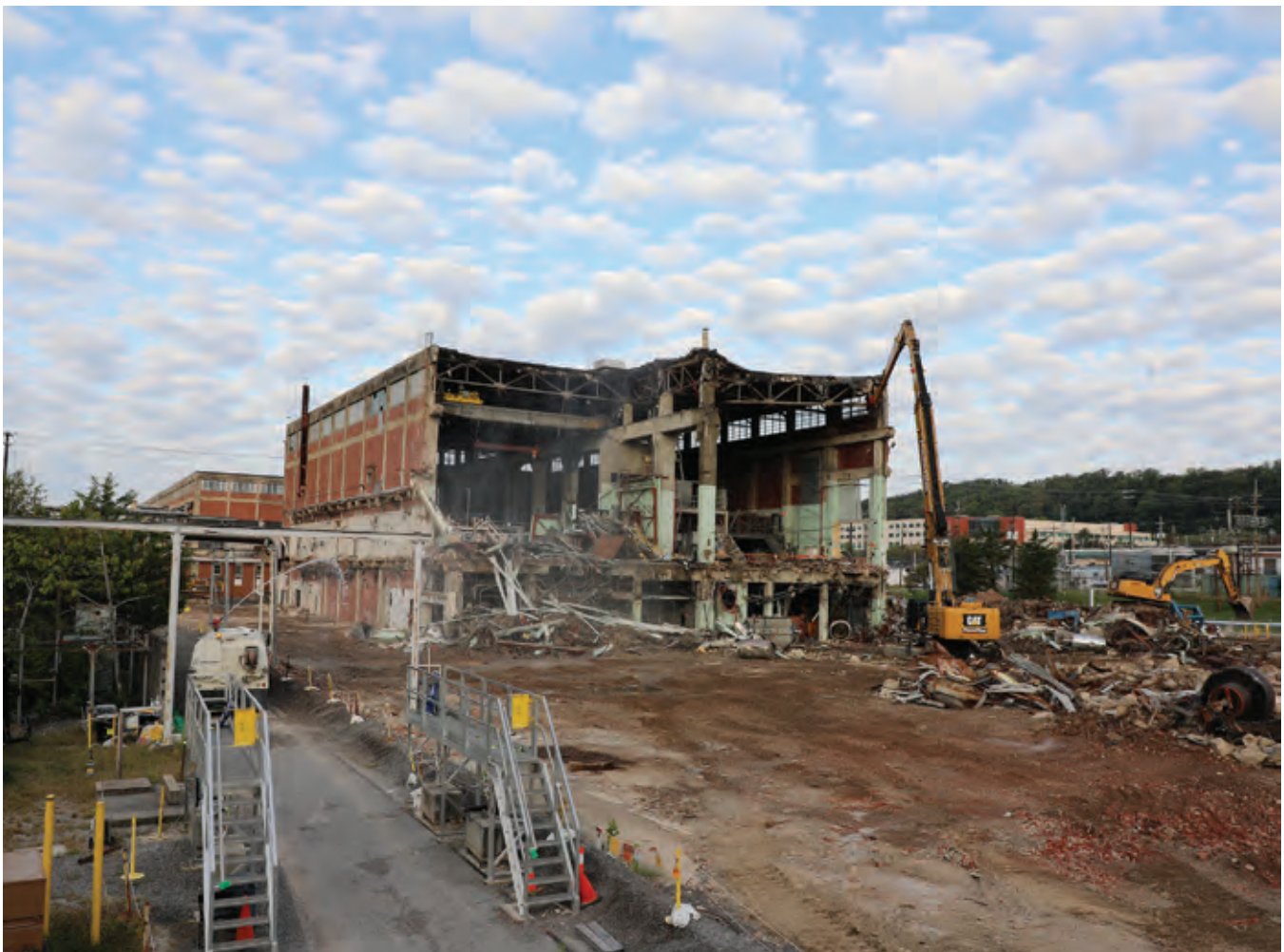
Demolition underway at the Alpha-2 Building
