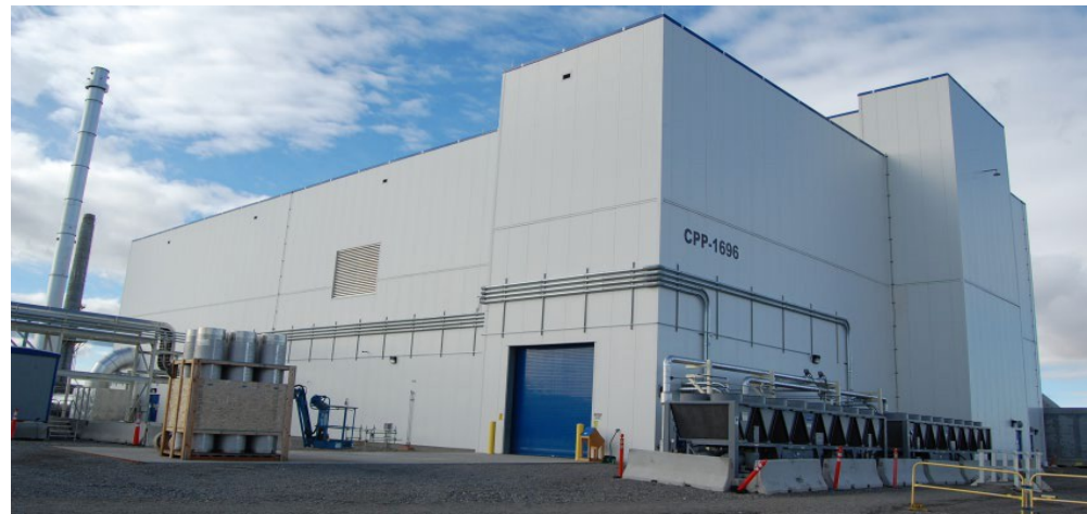
The Integrated Waste Treatment Unit
