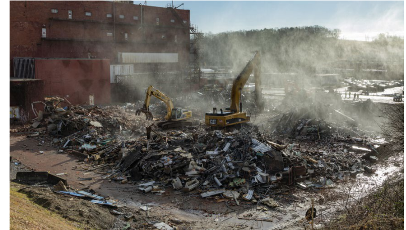
Crews finish demolition on Building 9210 at Y-12 National Security Complex
