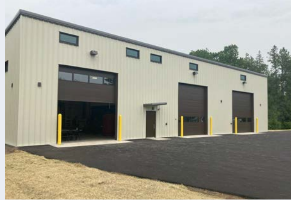
The biomass heating system facility for the Brookston Community Center was designed and constructed through a collaborative effort involving Tribal leadership, engineers, and local contractors. Photo by Joshua Gregory, Office of Indian Energy.
