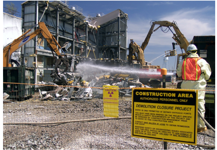
Remediation at the Fernald Preserve, Ohio, Site in 2006.
