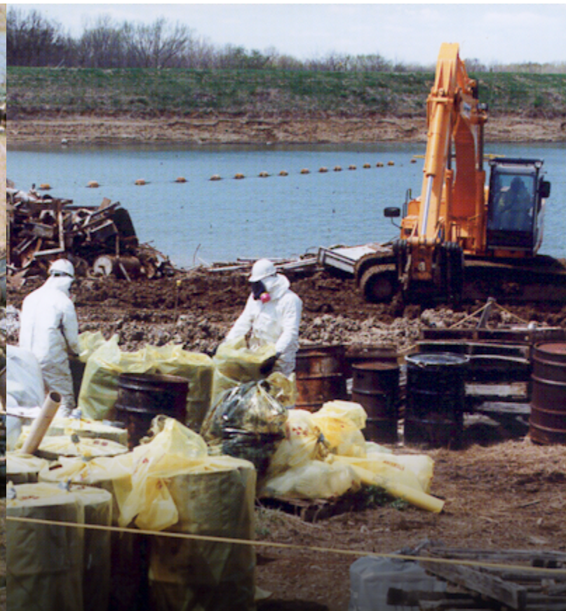
Barrels at the Weldon Spring Site, Missouri, raffinate pits required extensive cleanup during the Weldon Spring Site Remedial Action Project from 1987-2001.
