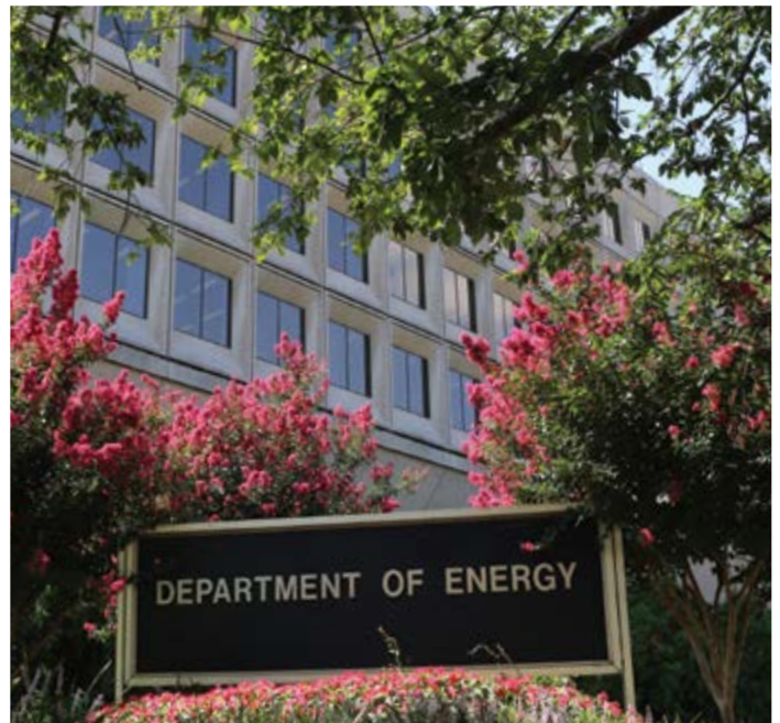
James V. Forrestal Building, Washington, D.C.
