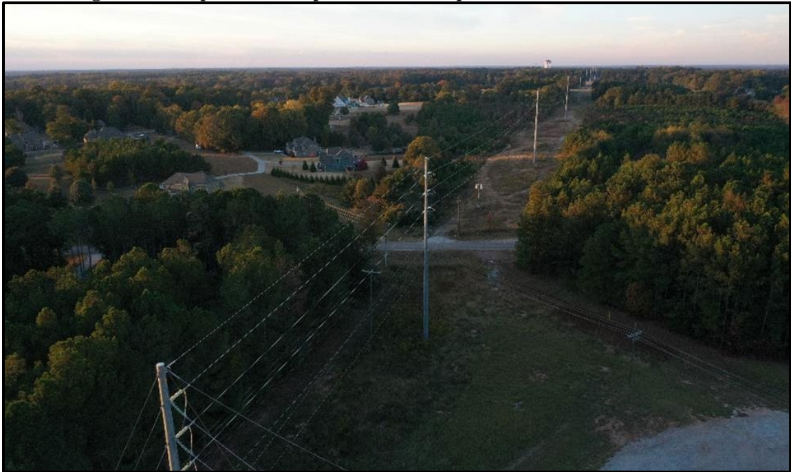
Figure 6.0 – Representative photo of a mono-pole concrete structure
