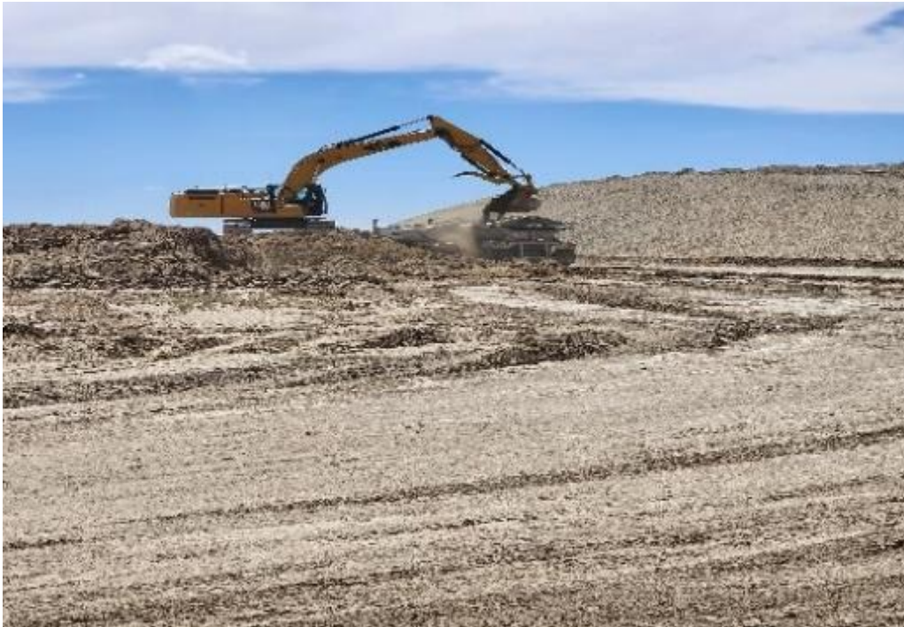
Photo 27. Loading Side Dump with Manco Shale for Interim Cover. August 2025
