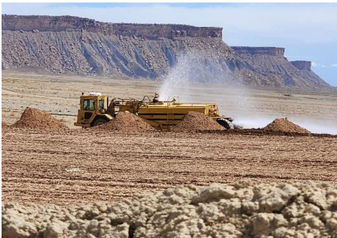
Photo 15. Water Wagon performing Dust Control. May 2025
