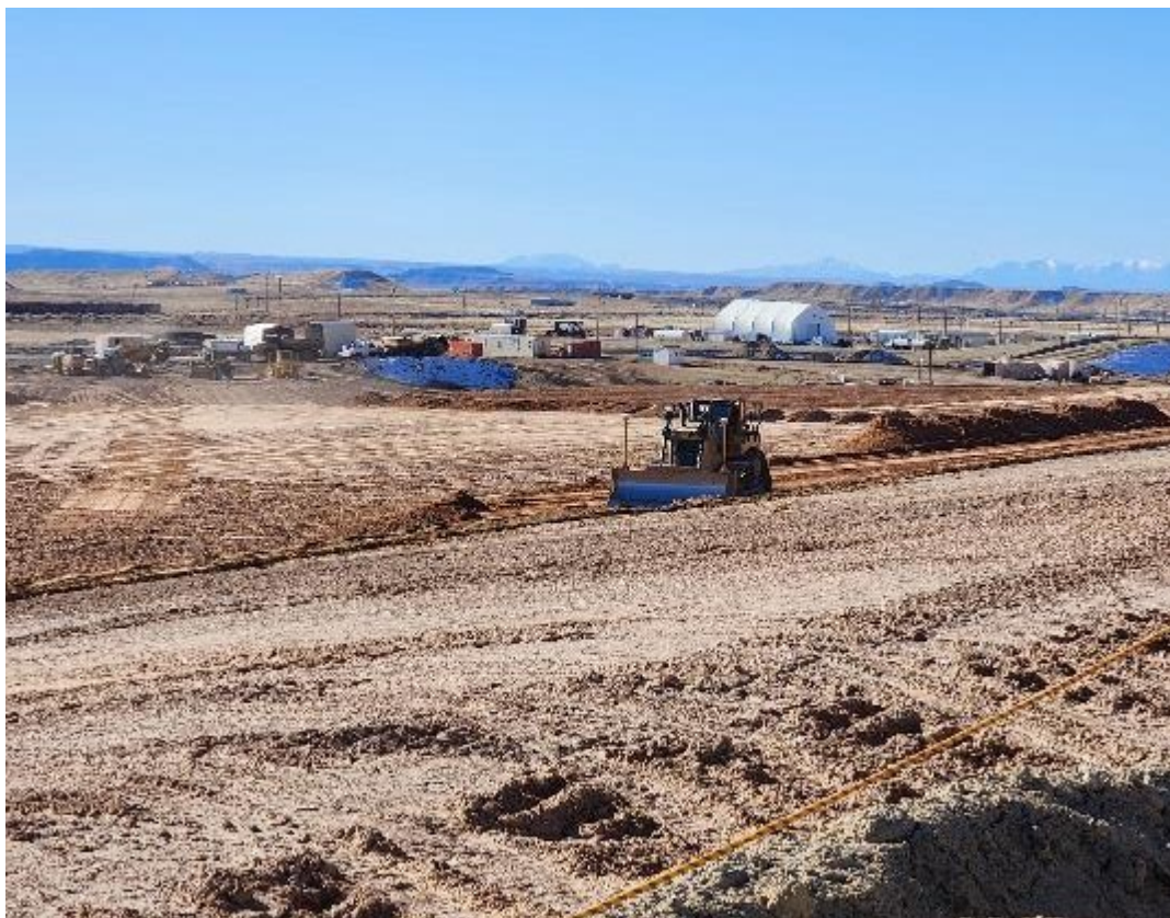
Photo 6. Dozer Placing Material on a Lift. December 2024
