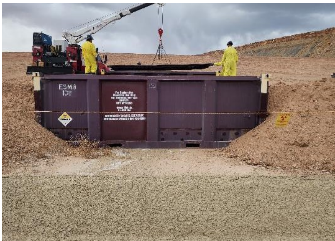
Photo 16. Lid Removal from One Trip Container. May 2025
