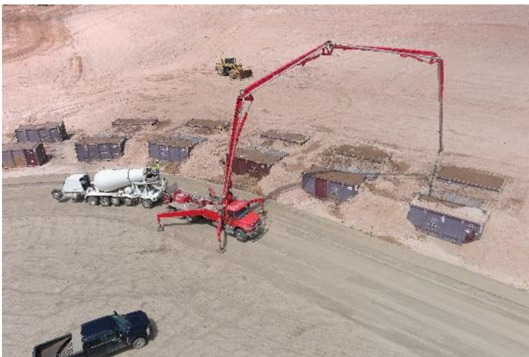
Photo 18. Filling One Trip Containers June 2025
