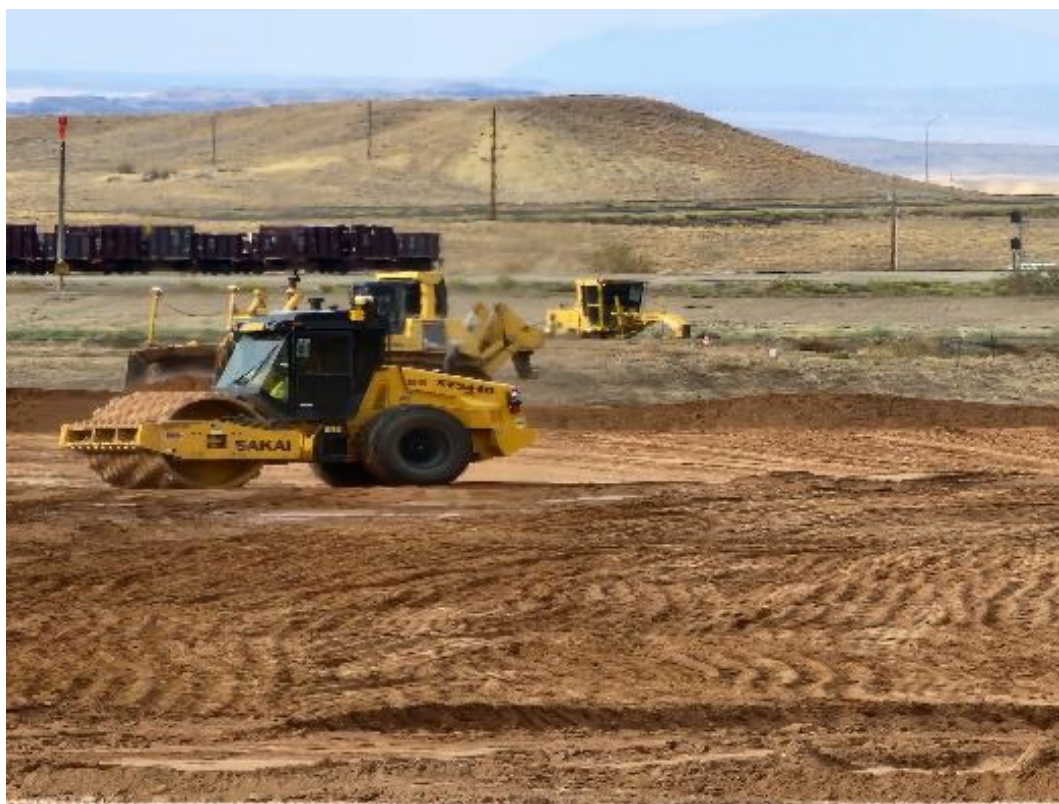
Photo 26. Compactor and Dozer Placing Material. September 2025
