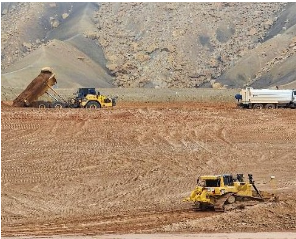
Photo 12. RRM Material Placement on Upper Lift. March 2025
