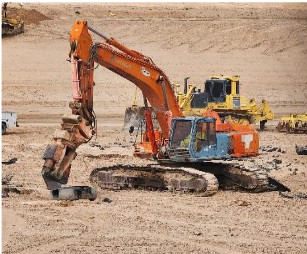
Photo 4. Size Reduction of Material Inside Disposal Cell. November 2024
