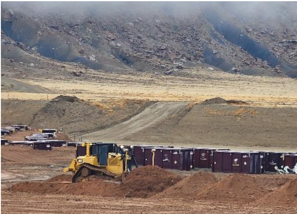
Photo 11. Dozer Placing RRM in proximity of One Trip Cans. March 2025
