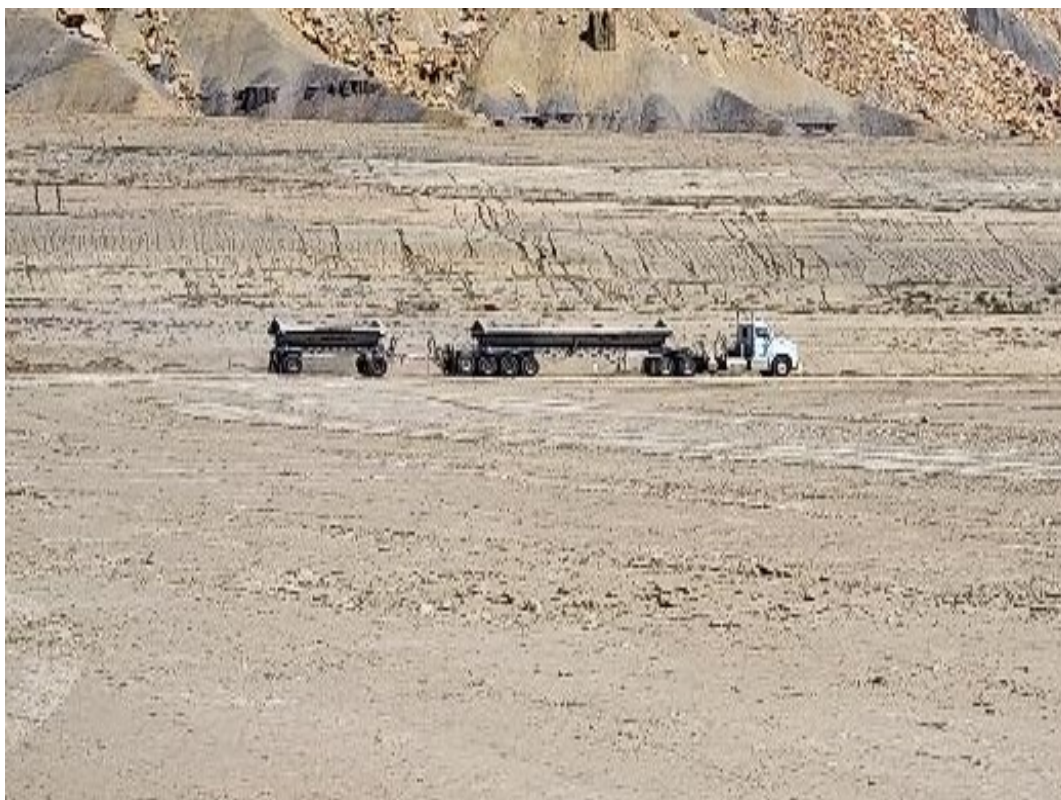
Photo 34. Side Dump for Protective Cover Placement. September 2025
