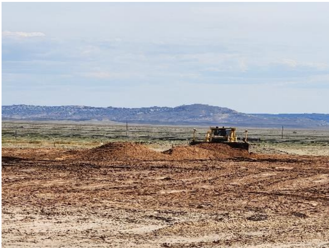
Photo 25. Dozer Placing Material on a Lift in the Cell. September 2025
