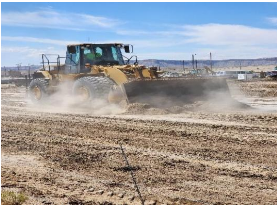
Photo 24. Loader Removing Top 6" - 8" of material from Fernald Rail Area. August 2025
