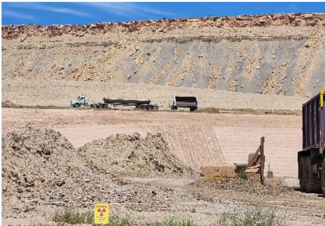
Photo 29. Side Dump and Pup Placing Manco Shale on Interim Cover. August 2025
