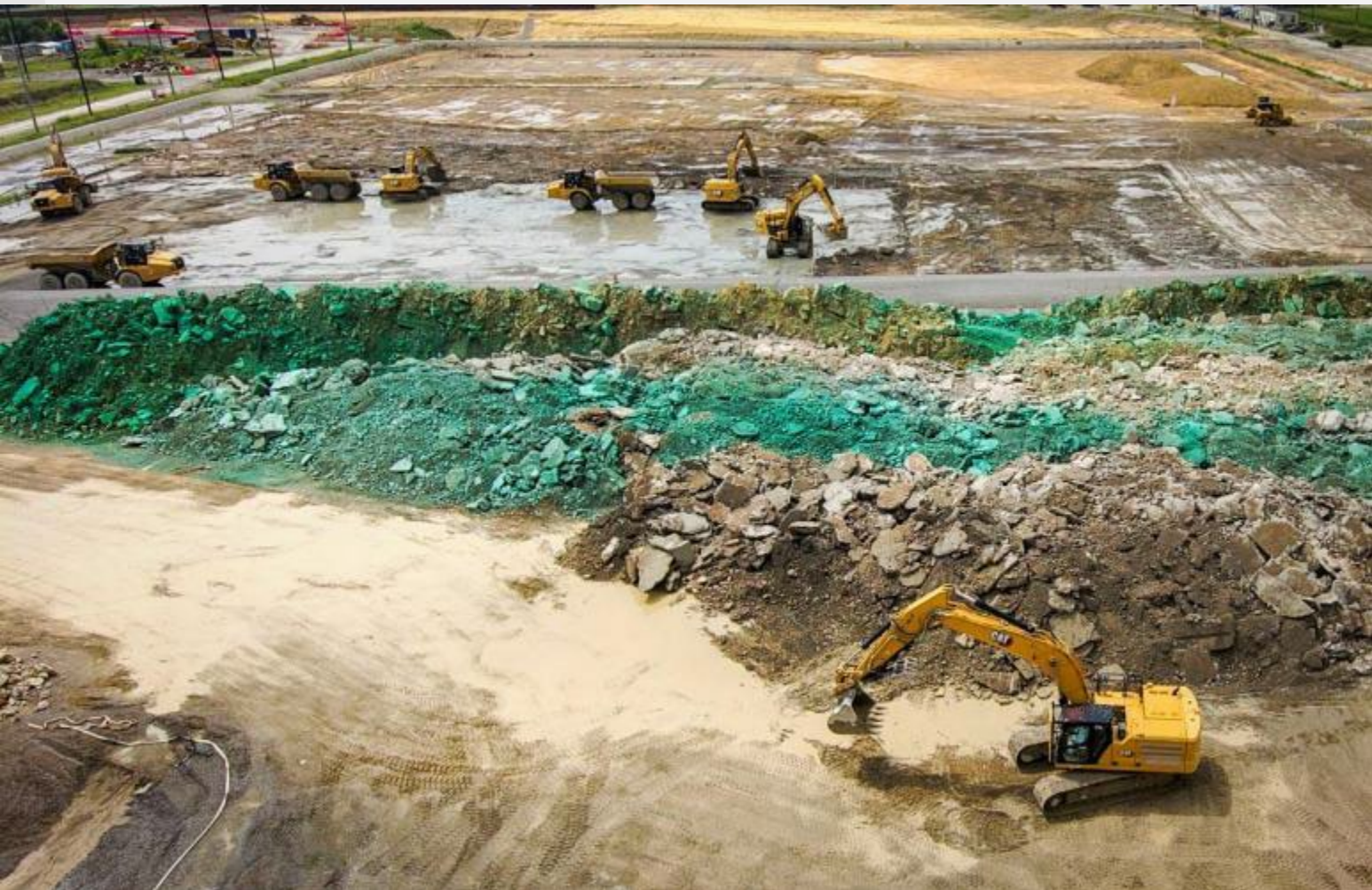
5-Unit Excavation Area
