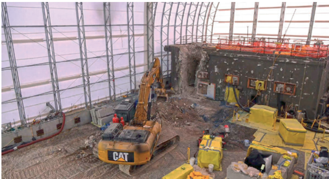
Workers demolish a portion of the final hot cell that was part of the former Radioisotope Development Laboratory
