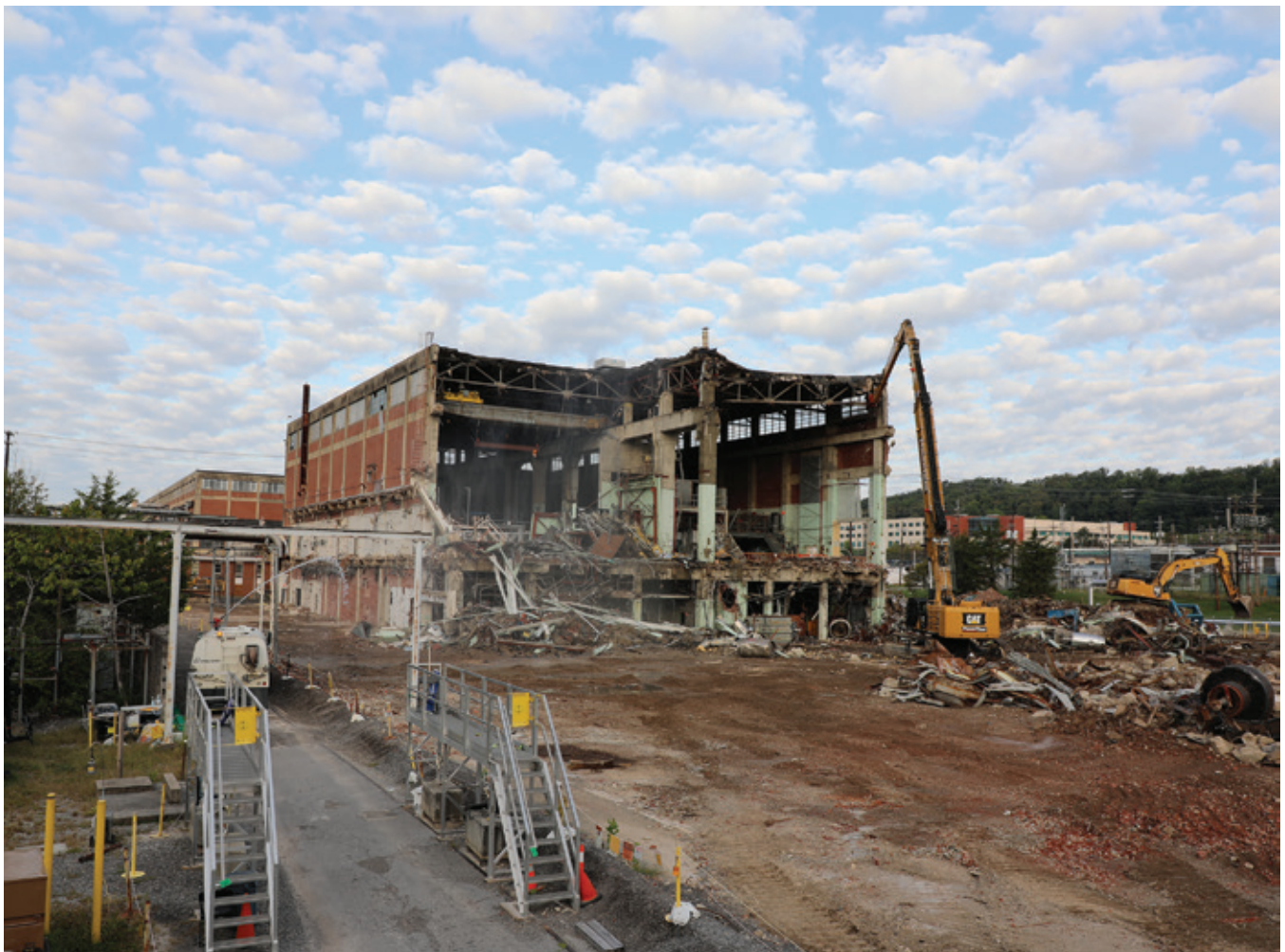
Demolition underway at the Alpha-2 Building
