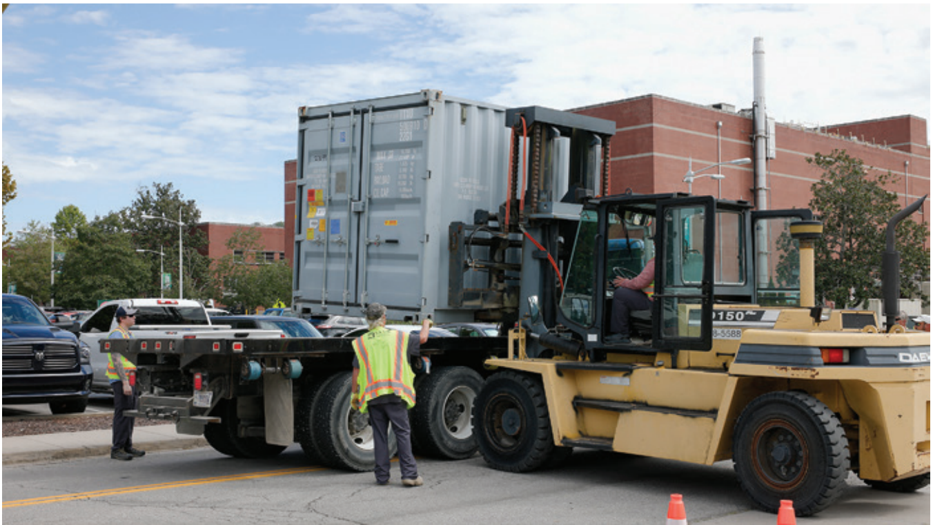
Workers remove a hot cell from Building 3038
