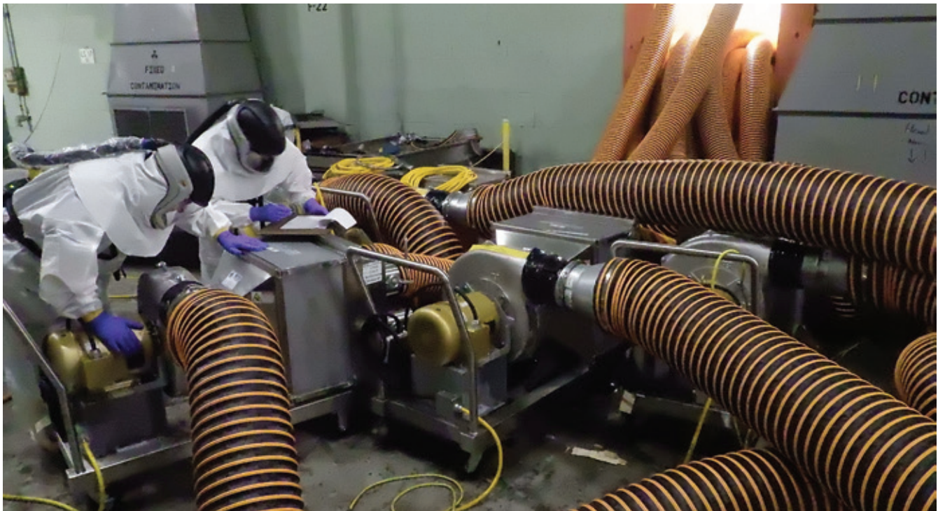
Air flow testing being conducted in Alpha-4
