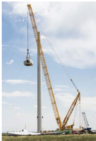
Figure 12. Crews lower the nacelle as part of the decommissioning of the 3-MW Alstom wind turbine at NREL's National Wind Technology Center. Photo by Dennis Schroeder. NREL 51733
