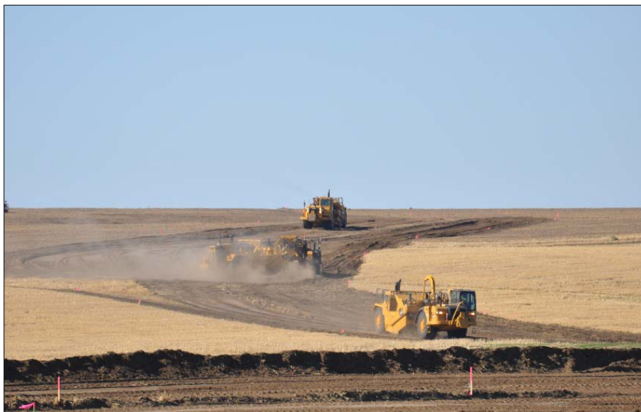
Figure 17. The construction of access roads for the Tucannon River Wind Farm near Dayton, Washington. Photo from Portland General Electric
