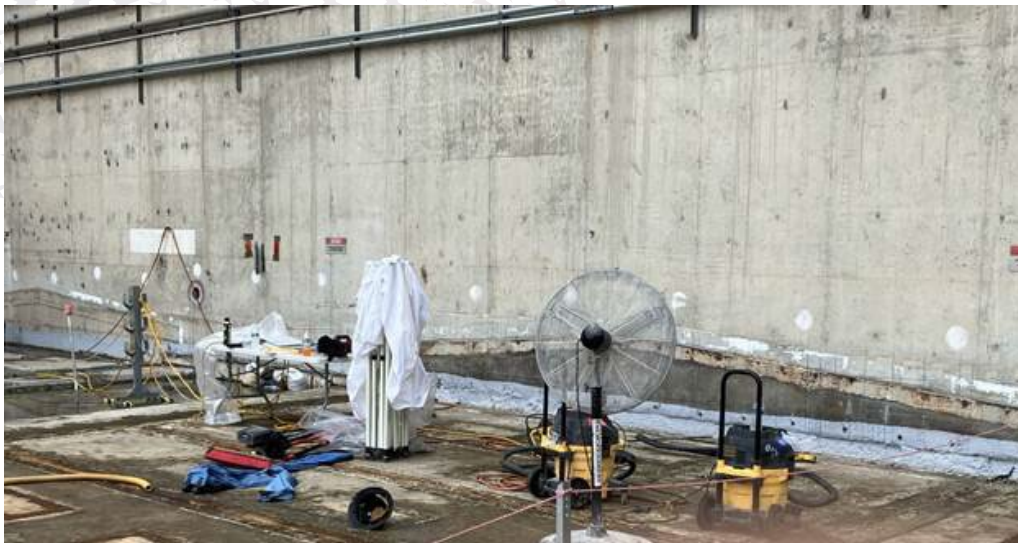
Figure 3.2-3: Outside Work Location (Handball Court) for Emplacement Holes
