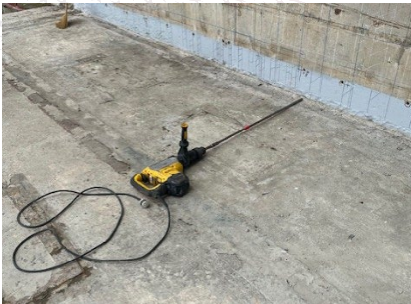
Figure 3.2-2: Longer Drill Bit for Horizontal Concrete Dowel Drilling
