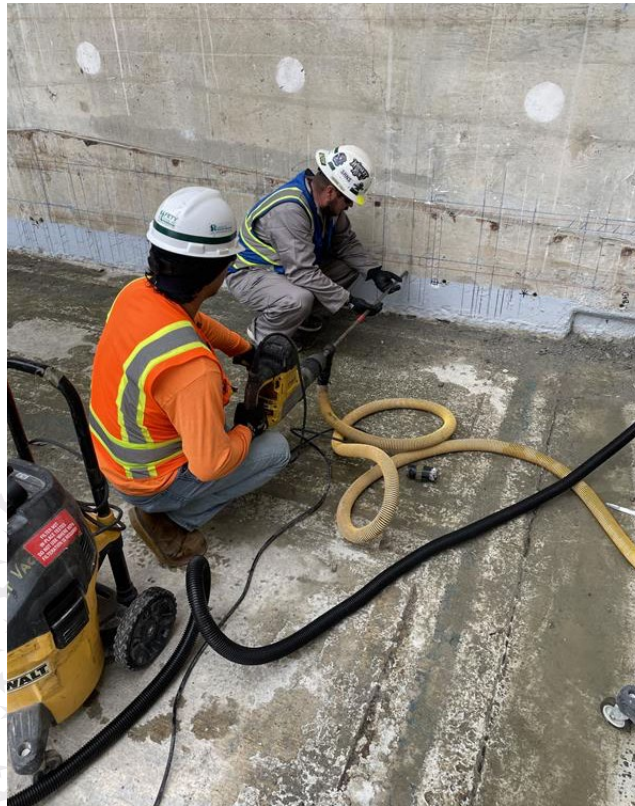
Figure 3.2-4: Reenactment of Ironworker Hand Guiding Horizontal Drill Bit
