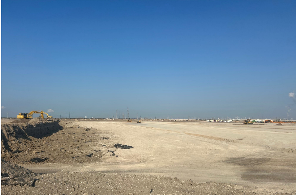
Photo 5: Trains 8 & 9 Site Preparation
