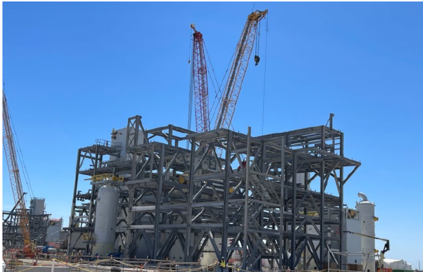
Photo 4: Train 7 Structural Steel
