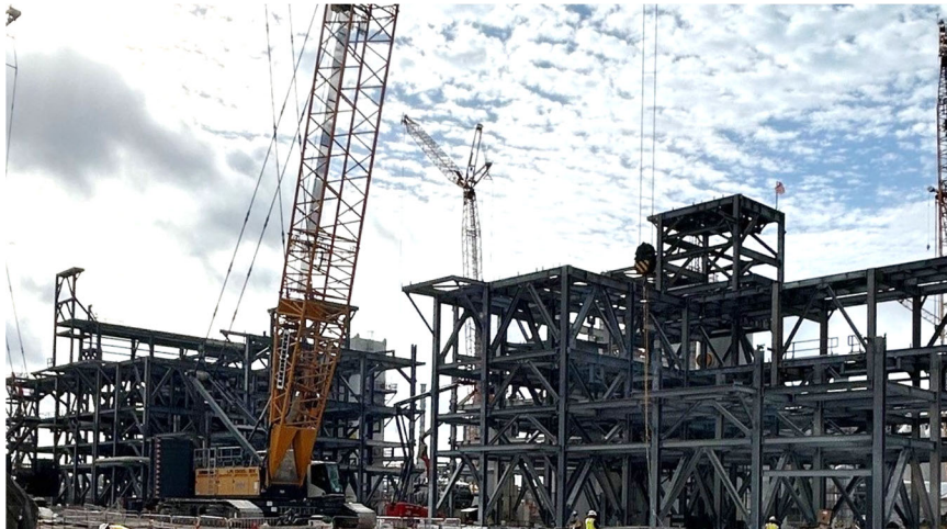
Photo 4: Train 6 Structural Steel
