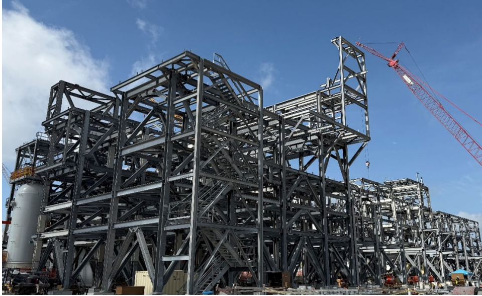
Photo 3: Train 7 Structural Steel
