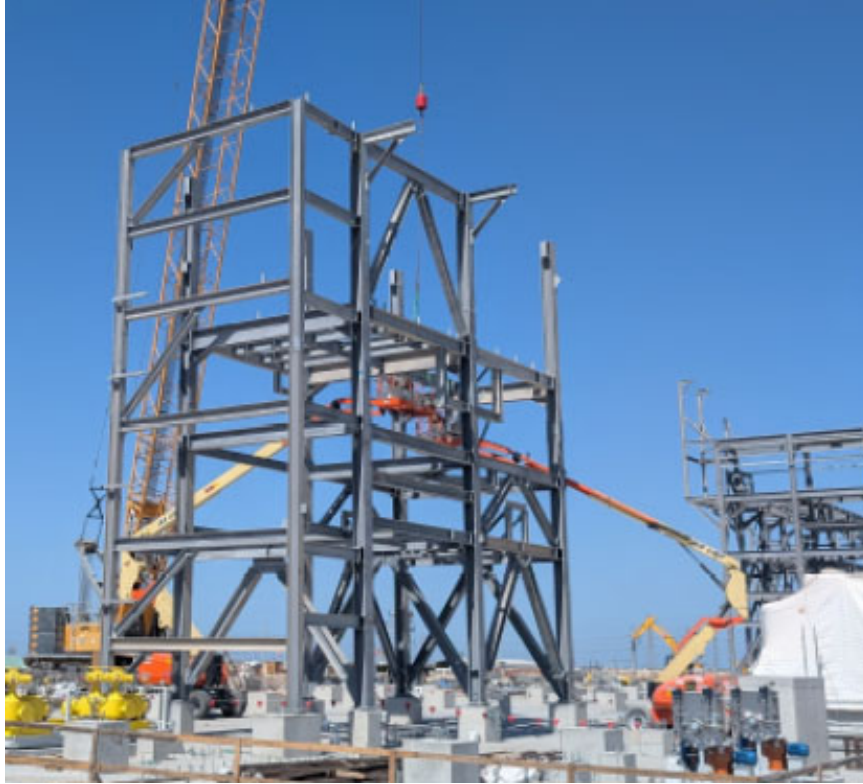
Photo 5: Train 7 Steel Erection
