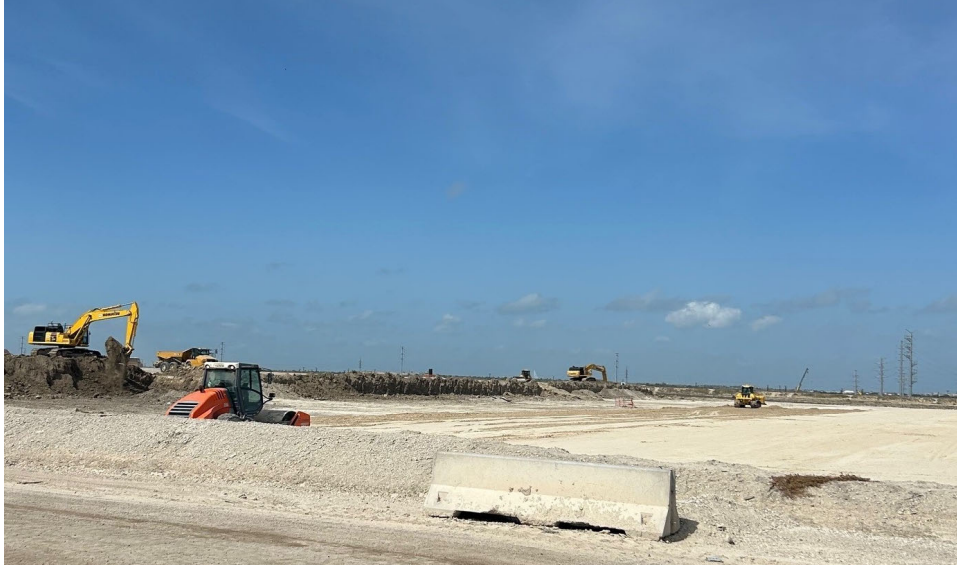
Photo 5: Trains 8 & 9 Site Preparation
