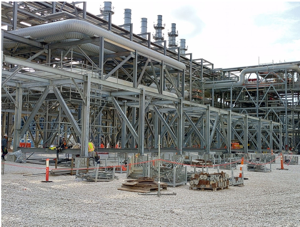
Photo 4: BOG 6 Structural Steel
