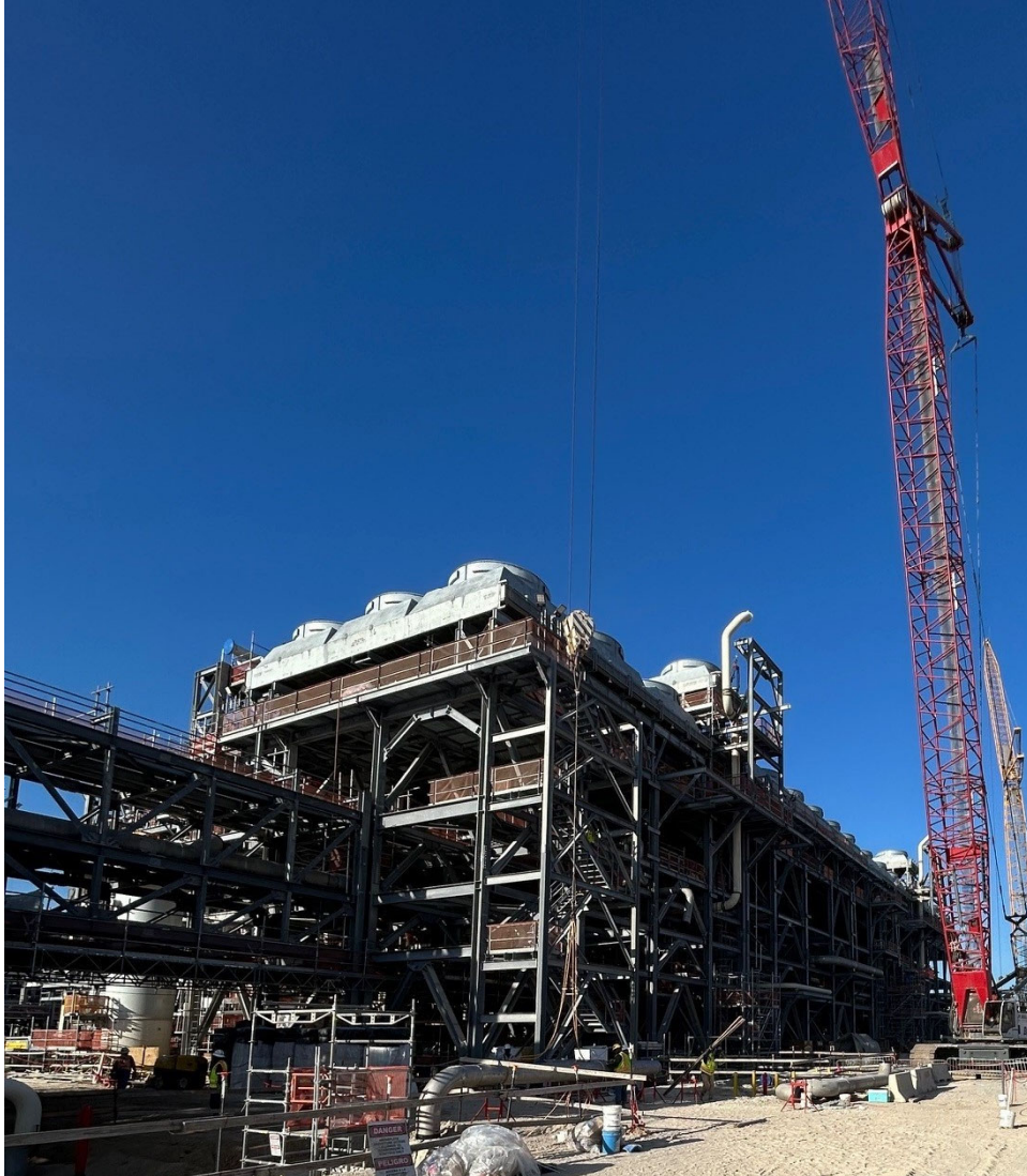
Photo 1: Train 5 Cryogenic Rack Area
