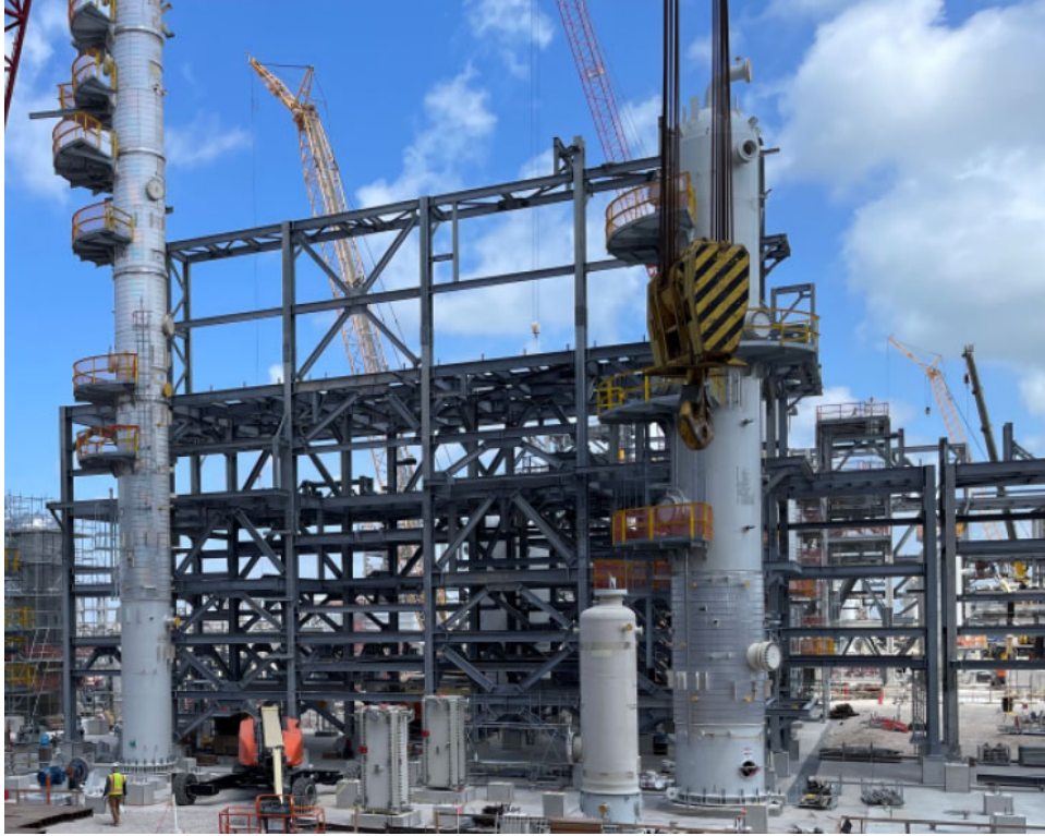
Photo 3: Train 6 Structural Steel
