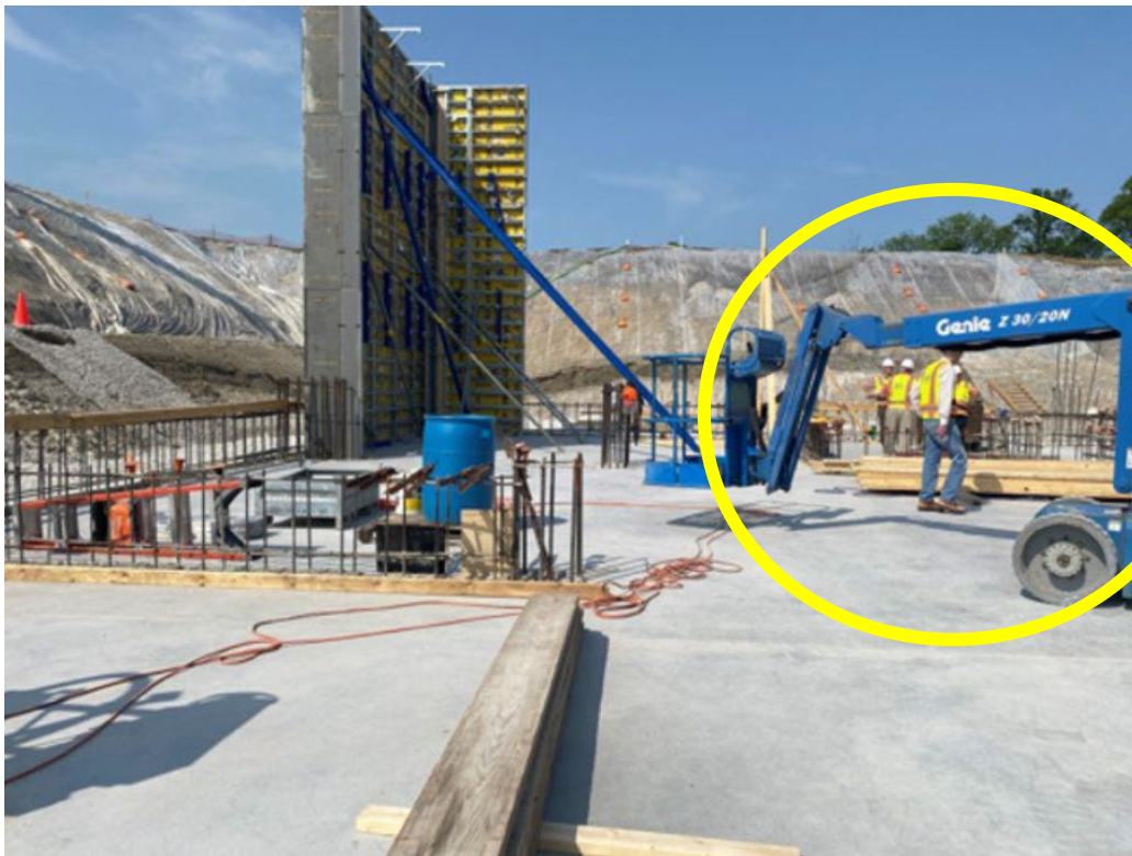
Figure 3: Aerial lift (Genie®)
