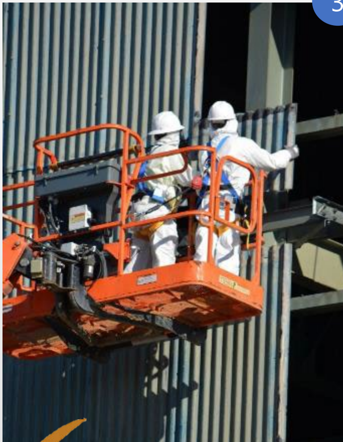
Transite (Asbestos) Removal
