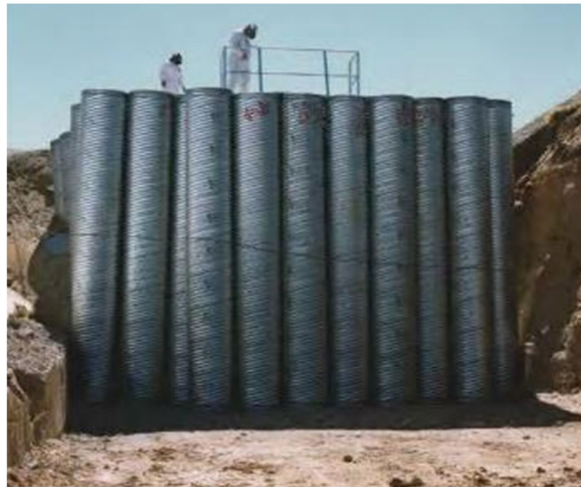
CMPs were emplaced vertically at TA-21 until 1986
