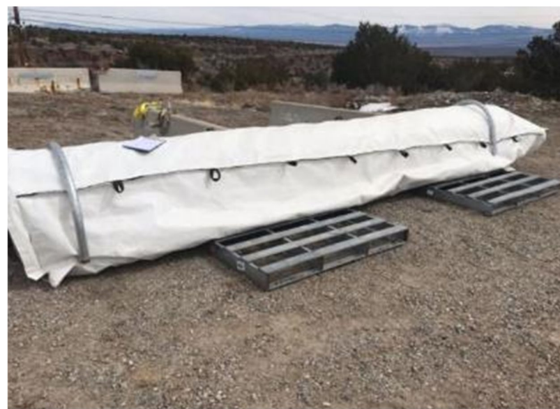
CMPs placed into IP-1 bag after removal from above Pit 29 and prior to placement on Pad 10
