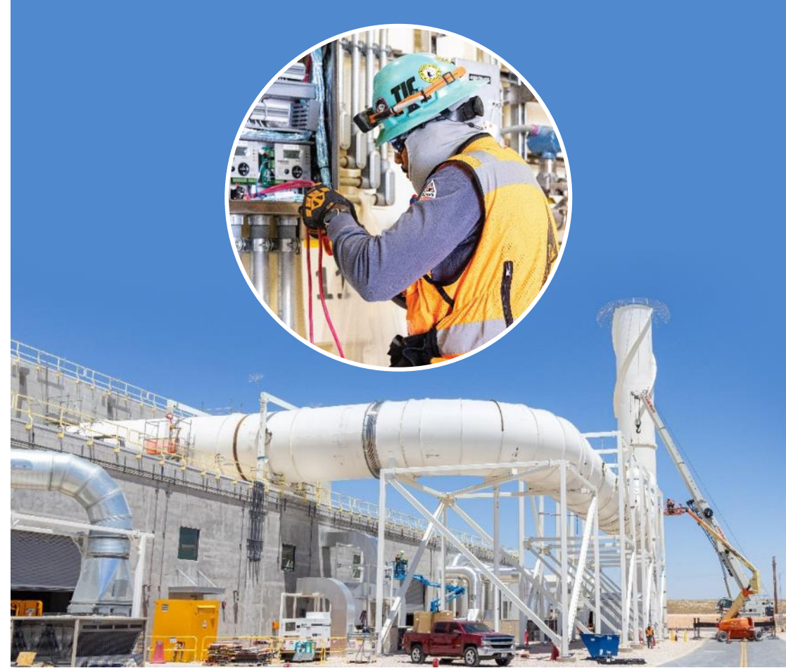
Above: Equipment testing during SSCVS commissioning Below: SSCVS final large duct work installation
