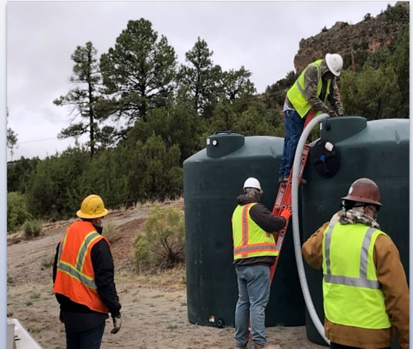
ER Well Drilling Water
