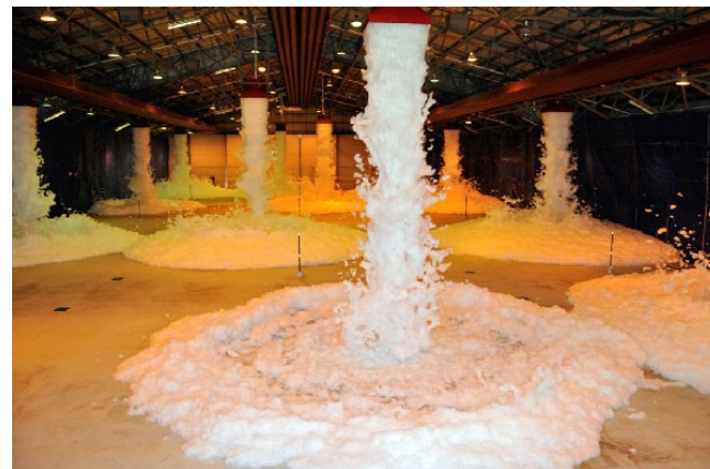
Example of AFFF in an industrial setting for illustration purposes only
