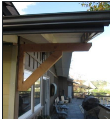
Example Gable Overhang Bracing Using Gallow Brackets ( Mahan 2014 )
