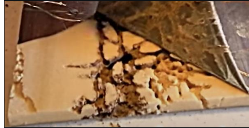
Example of foam board insulation that termites have tunneled through (Campbell Law, P.C. 2013).
