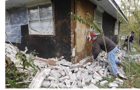
Earthquake Fragility of Masonry Veneers ( Khosravikia et al. 2020 )
