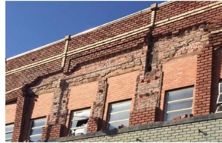
Earthquake Fragility of Masonry Veneers ( Khosravikia et al. 2020 )
