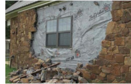
Earthquake Fragility of Masonry Veneers ( Khosravikia et al. 2020 )
