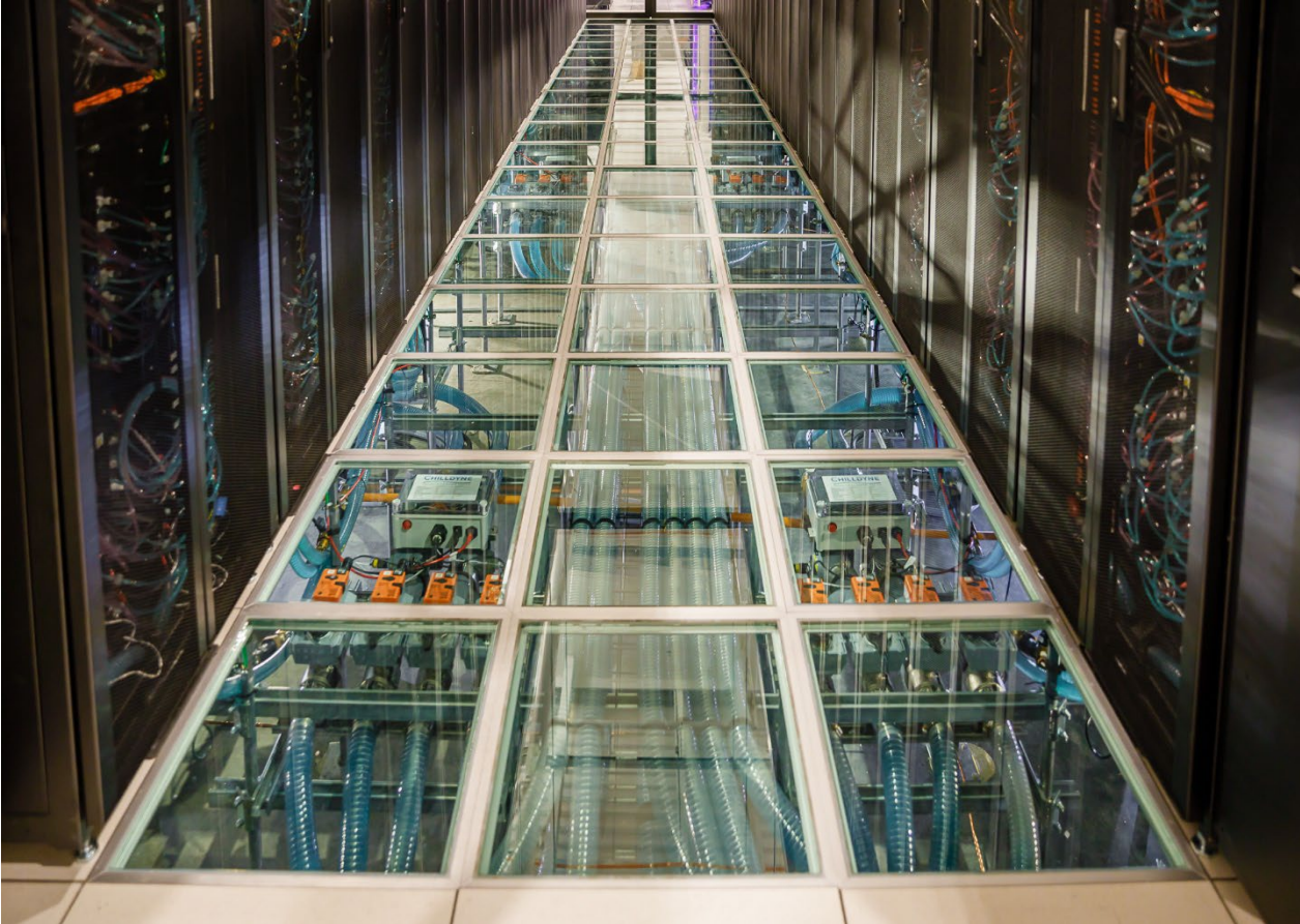
Attaway's negative pressure cooling system (70% liquid)
