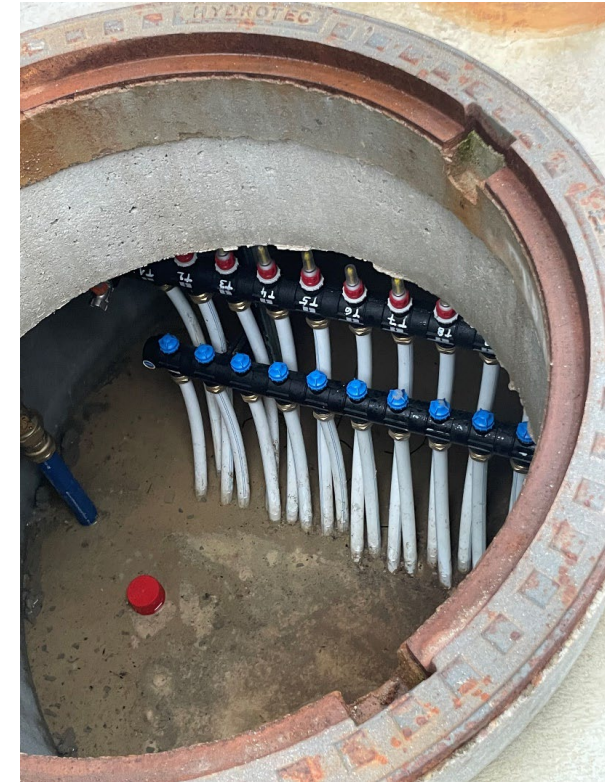
Tie-in of ground heat exchanger system at central plant
