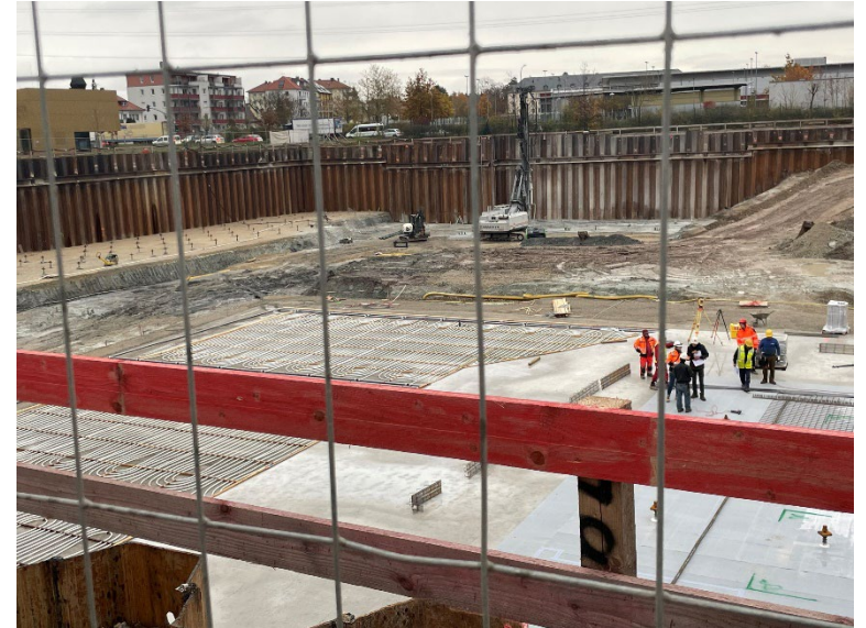
Horizontal GHE installed to serve district energy system. Photo courtesy of Matt Mitchell.
