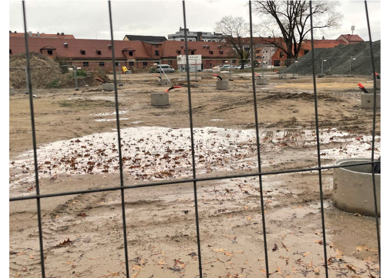
Vertical GHE wells installed to serve district energy system before tie in. Photo courtesy of Matt Mitchell.
