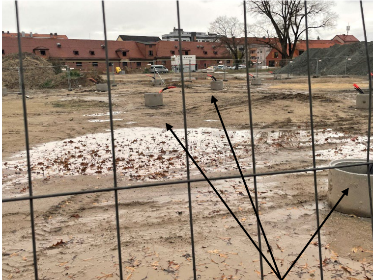
Locations for pipe tie-ins to vertical wells before tie-in. Concrete “collars” are temporary.
