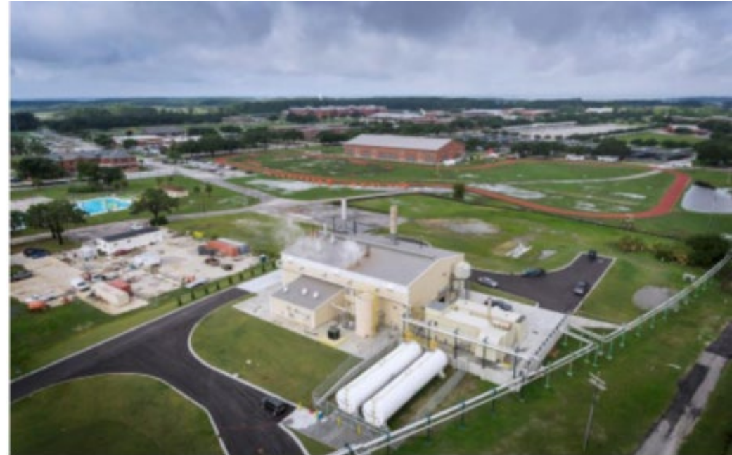
MCRD's new central plant with microgrid and island mode capability providing 3.5 MW of electric and the full steam load required by MCRD Parris Island. Photo courtesy of Business Wire
