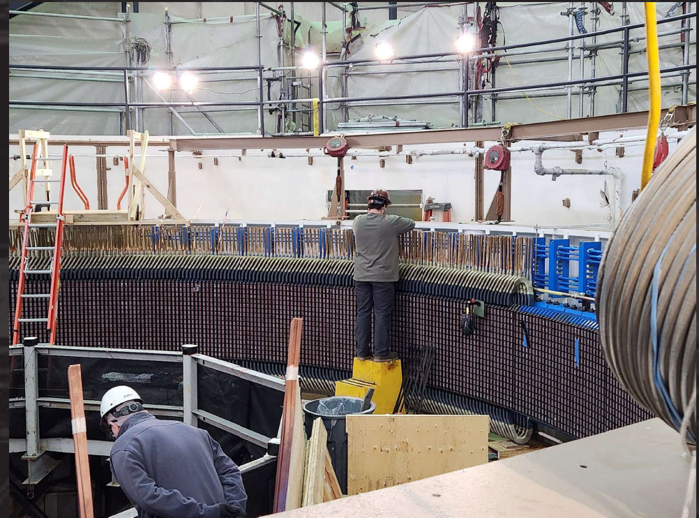
BAR TG, Stator Coil Installation
