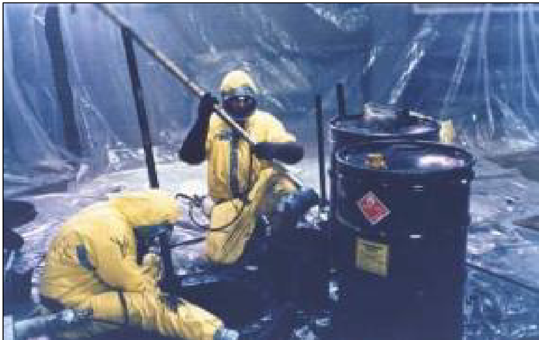
Figure 11-2. Removing Sludge and Placing It in Drums at the Chicago North Site (DOE Digital Archive)
