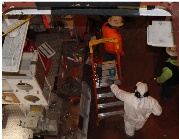
Idaho Cleanup Project crews perform deactivation activities at the Aircraft Carrier 1st Generation Westinghouse prototype, including hazardous materials removal, prior to beginning demolition of the facility.
