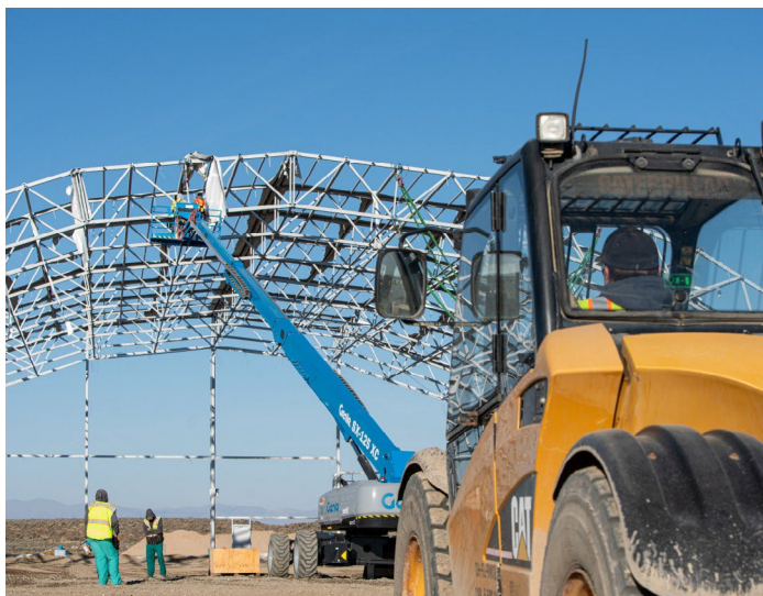
Idaho Cleanup Project demolition crews prepare to pull down a large, steel Accelerated Retrieval Project enclosure at the Idaho National Laboratory Site.
