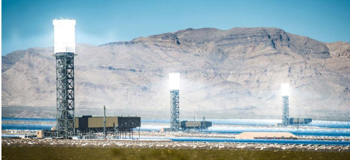
**Figure 6-2. Ivanpah water/steam receivers**
