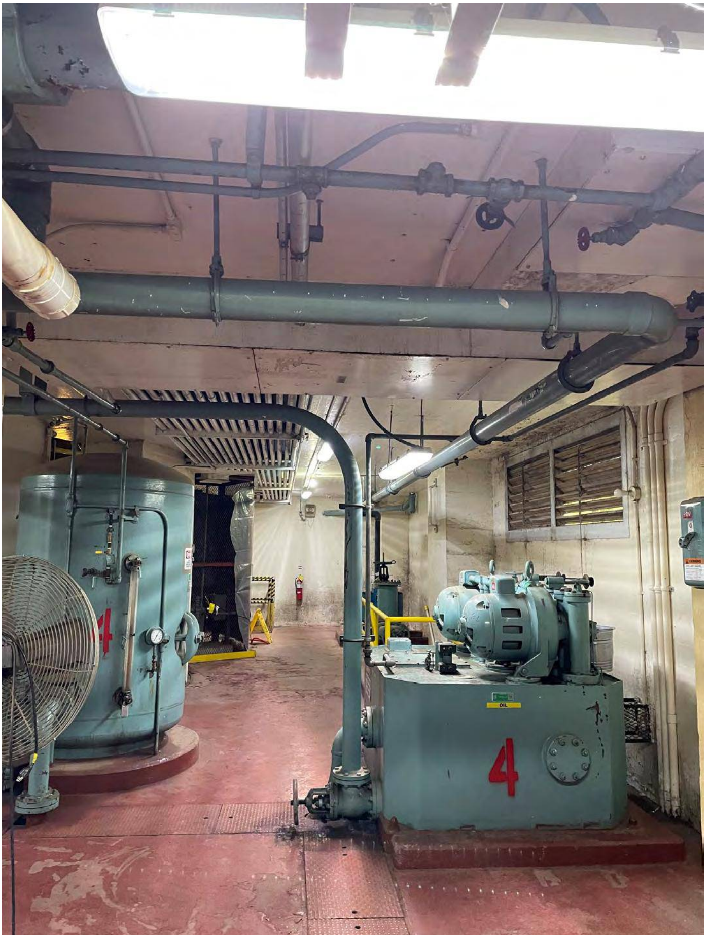
Figure 4. Photograph showing turbine floor.
