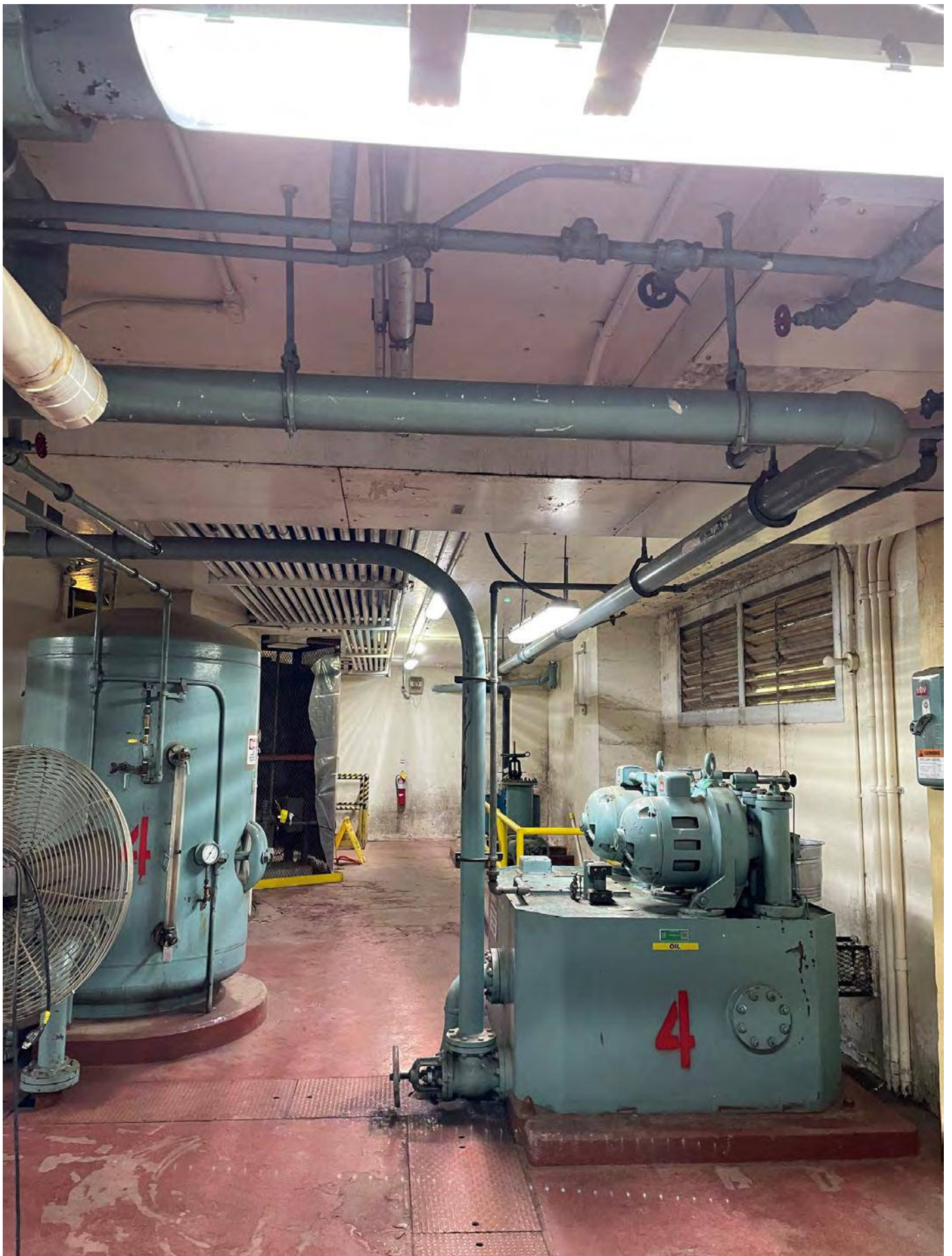
Figure 4. Photograph showing turbine floor.
