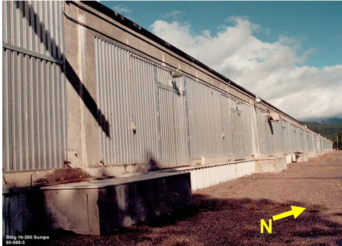
Back of HE machining building TA-16-260 showing HE sumps & blowout walls – sumps discharged to single outfall to northeast of building
