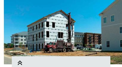
Geothermal heat pump drilling at a new housing development in Norton Commons, North Village, Kentucky. *Photo by Norton Commons*
