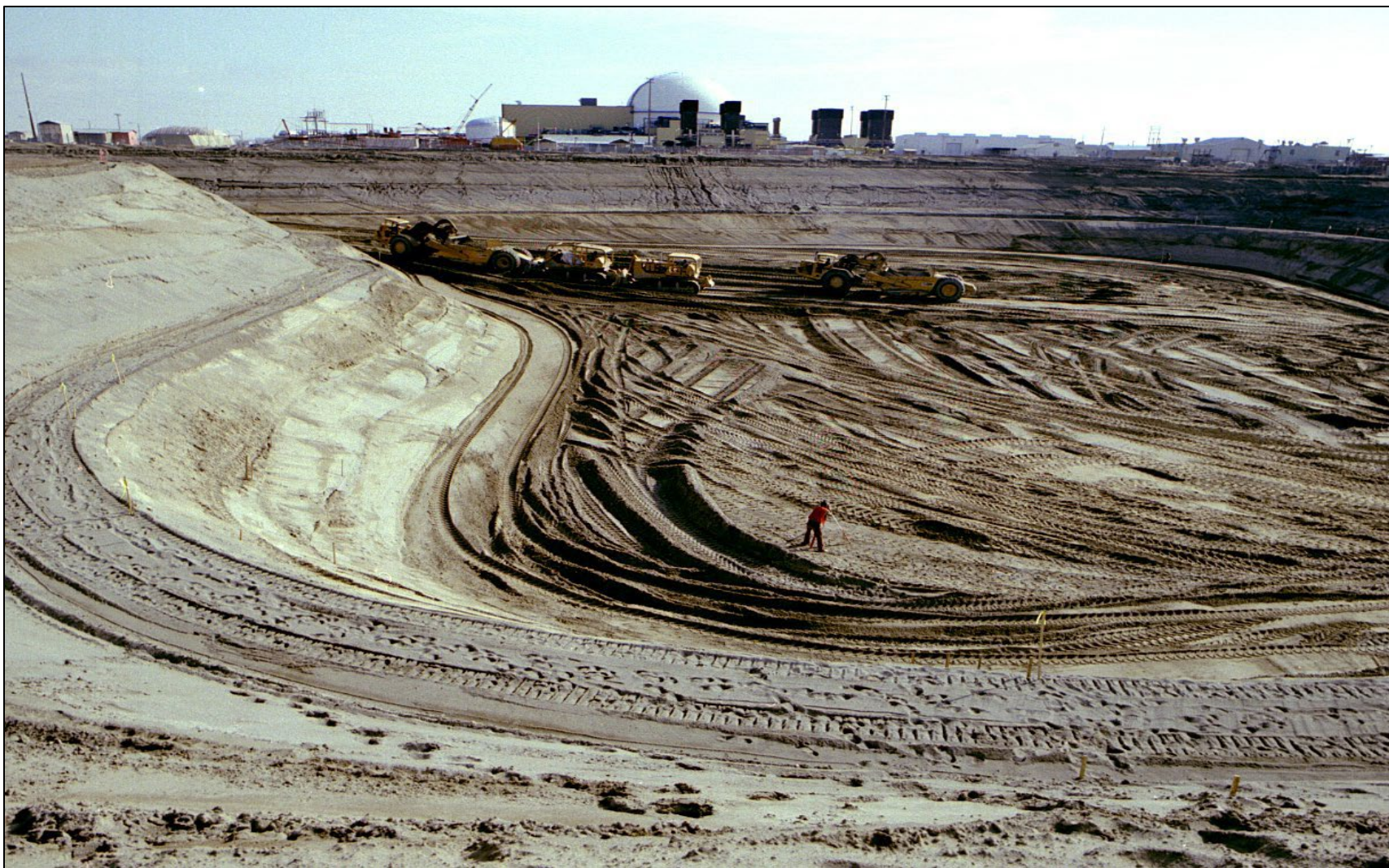
Figure 6 - FMEF Excavation for Minus 35 Feet and Minus 17.5 Feet Elevation Structures – Hanford Site 400 Area
