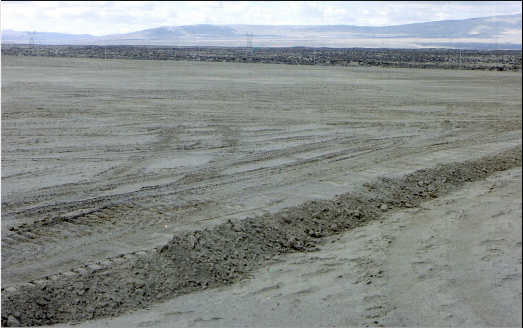
Figure 5 – Initial Clearing and Grubbing of FMEF Construction Site – Hanford Site 400 Area
