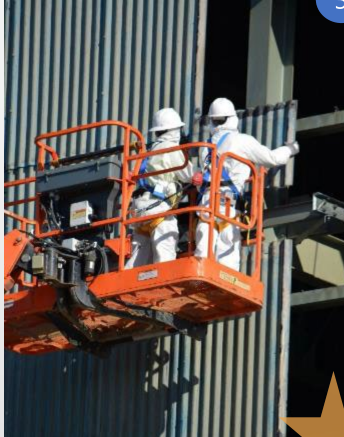
Transite (Asbestos) Removal
