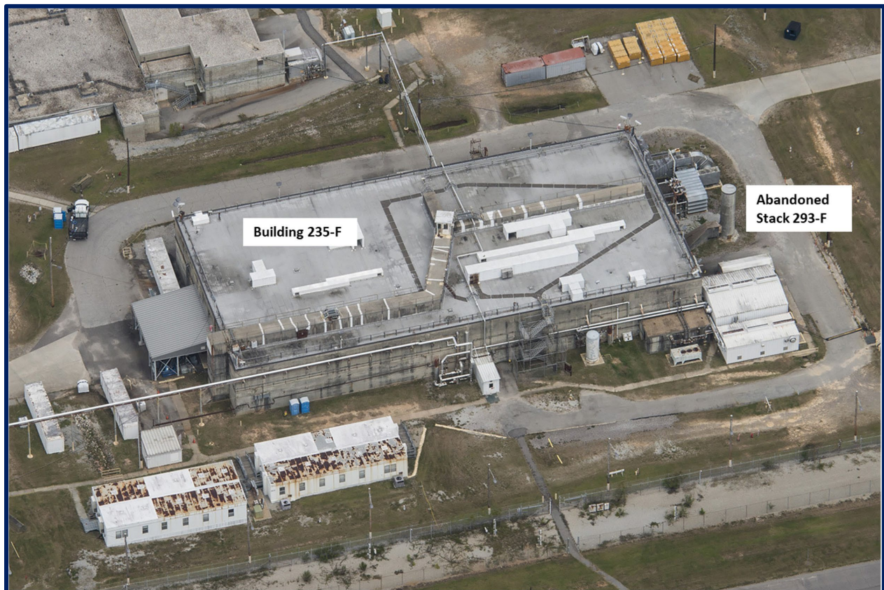
Figure 1. Building 235-F – Savannah River Site (SRNS-RP-2020-00444).
