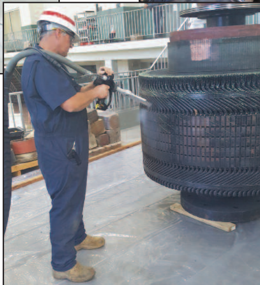
Allatoona generator rotor removal (top left) prior to stator winding (above) and excitation (left) electrical component carbon dioxide blast cleaning.
