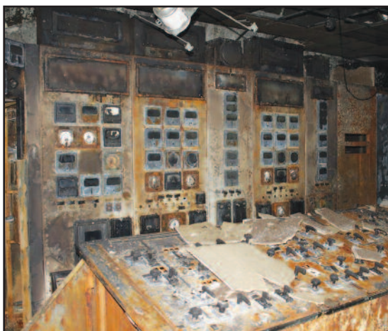
Allatoona control room (above) and generator floor (below) after the fire. New switchyard breakers were being stored on the generator floor prior to installation.
