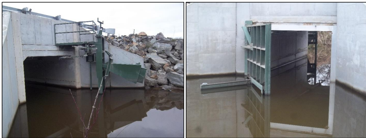
Figure 2-2: Example concrete box culvert with automated tide gate proposed for the Auto Tour Route and Deep Creek Breach.
